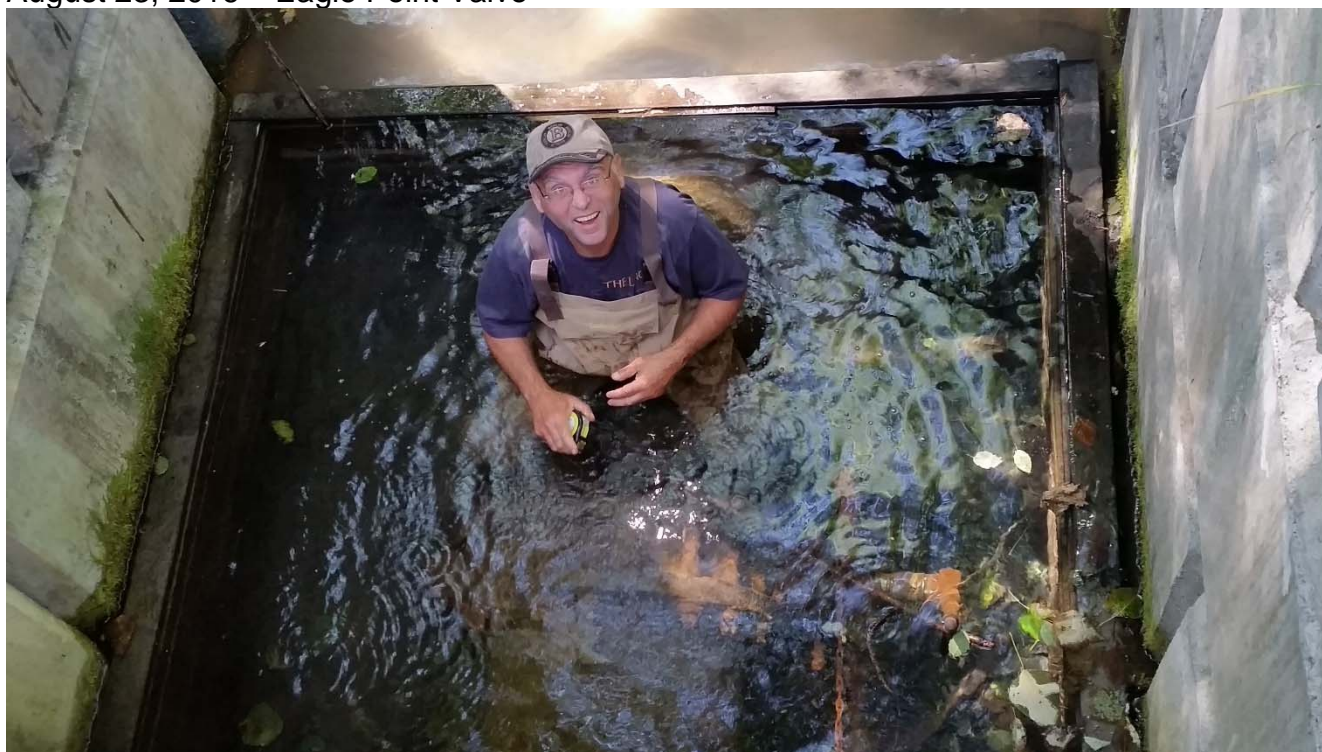
Looking down into Eagle Point Valve (prior to upgrade)
