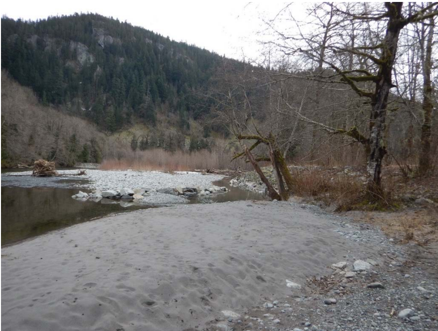
Mykiss Channel (east side of Bailey bridge – facing downstream on Cheakamus River) – removal of log jam and woody debris build-up
