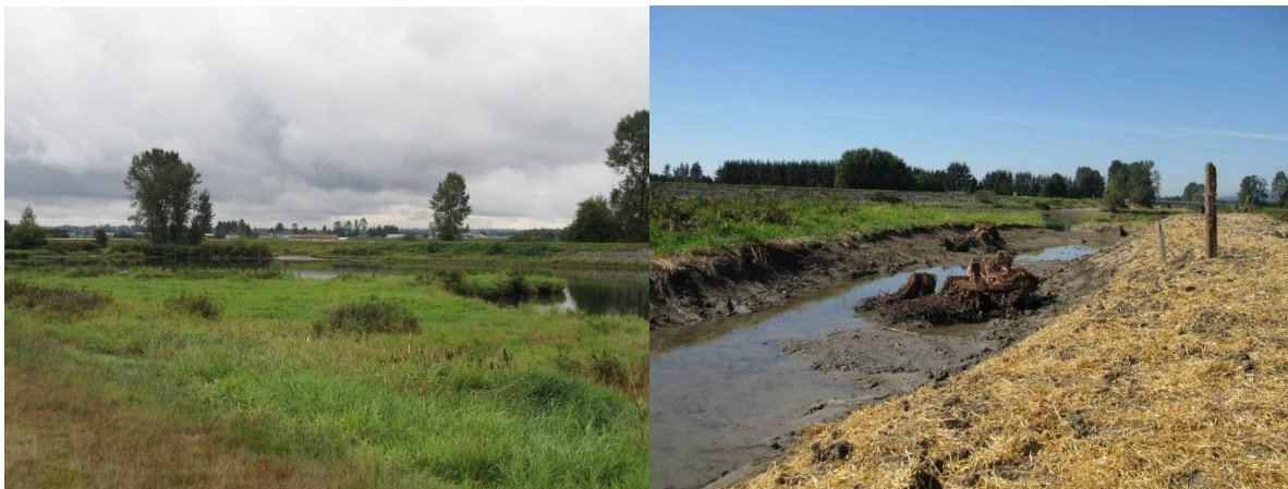
Figure 5. Harris North restoration site pre-restoration (left, view east) and post-restoration (right, view west) showing anchored large wood within excavation to create tidal marsh.
