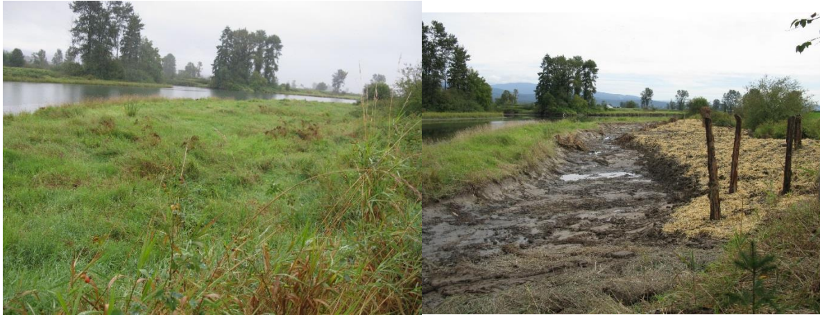
Figure 4. Harris South restoration site pre-restoration (left) showing low bench 95% covered with reed canary grass, and post-restoration (right, view west) showing excavation to create tidal marsh and anchored large wood.
