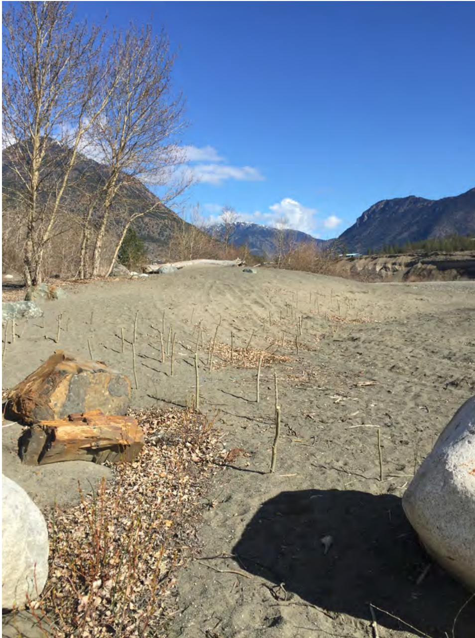
Figure 19 Boulder cluster and cottonwood cuttings at B18 29 March 2017
