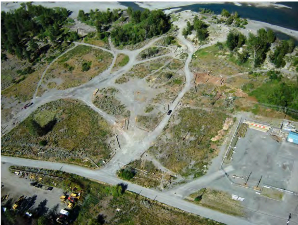
Figure 2 Section of upland bench – compacted soils, roads and invasive species prevalent on site 11 July 2008
