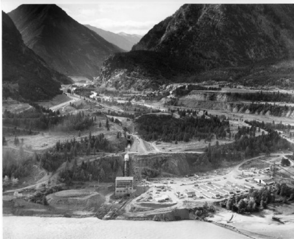
Figure 1 Cayoosh Canal and Forebay Construction 1950s
