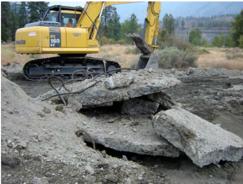
Figure 6 Concrete slabs being removed August 2009
