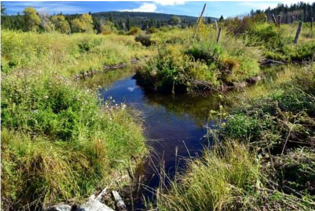
Here is one of many emergent wetlands built to manage stormwater runoff near Logan Lake, British Columbia.
