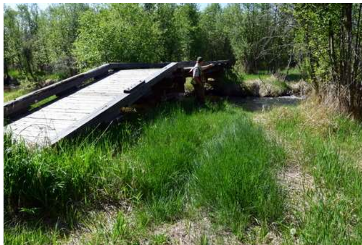
Here is the existing bridge over Cherry Creek
