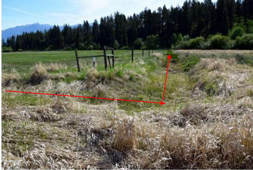
Deep ditches, like the one shown, were dug to divert runoff from Cherry Meadows.
