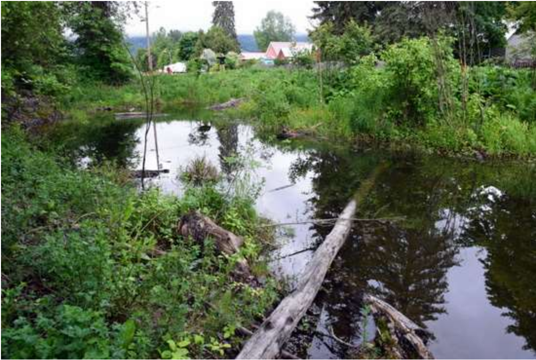
Emergent wetland built for treating stormwater at KP Park, Salmo, British Columbia
