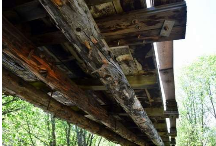
The existing bridge is supported by small diameter logs
