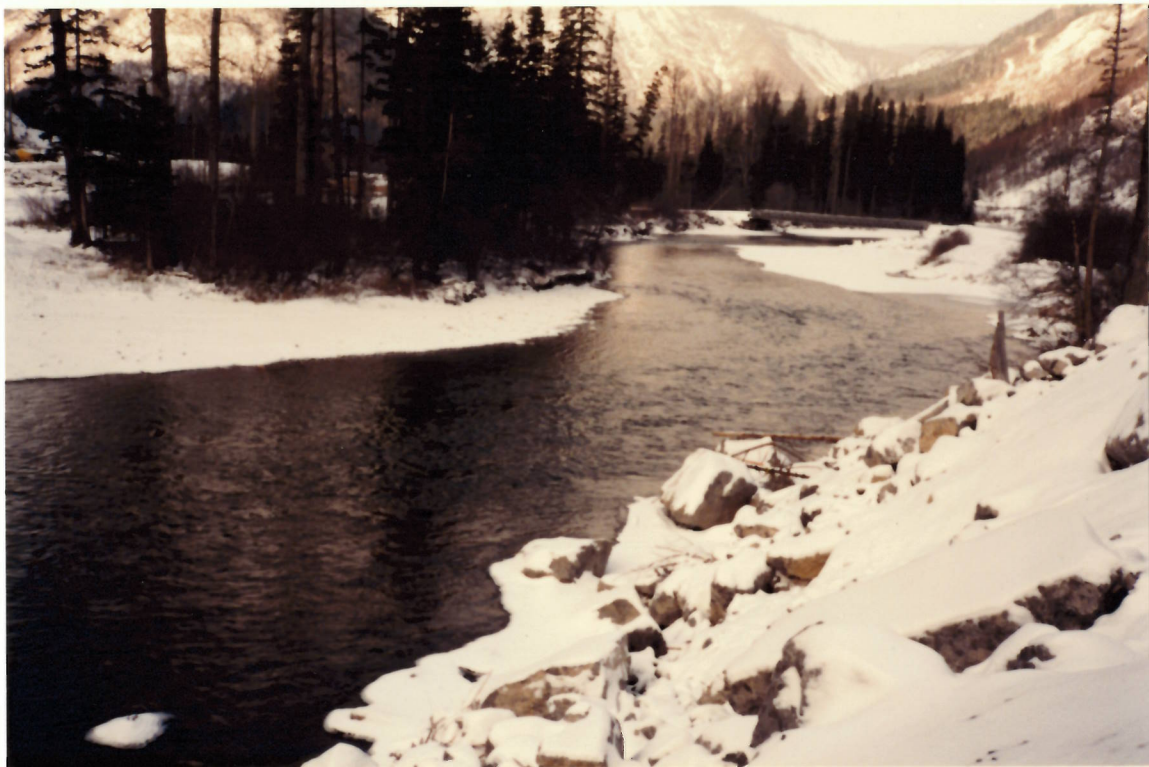
Figure 7 Example of displaced rip-rap in the upper Pine River.
