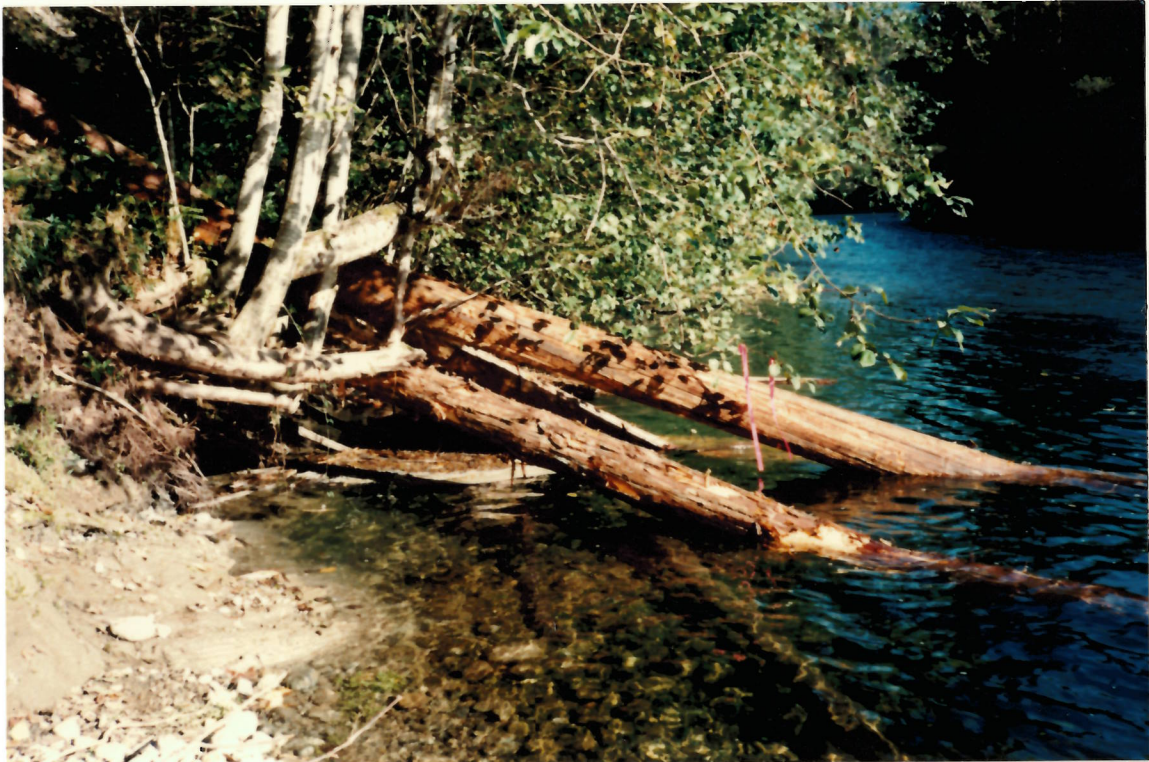
Figure 6. Example of bank LOD structures installed in the Cowichan River, 1991.
