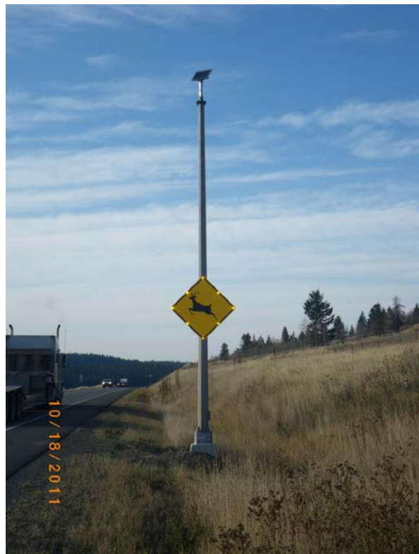
Figure 9. LED-enhanced deer collision warning sign, located on Highway 97 north of 100 Mile House (G. Hesse).
