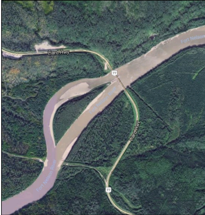
Figure A2: Air photo view of the Fort Nelson River Bridge crossing on Highway 77. Note the broad floodplain area south of the bridge likely underlain by sands and gravels of the Fort Nelson River aquifer.
