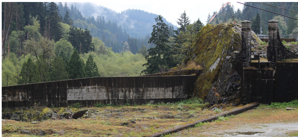
Figure 12. Photograph of the West End of the Spillway.
