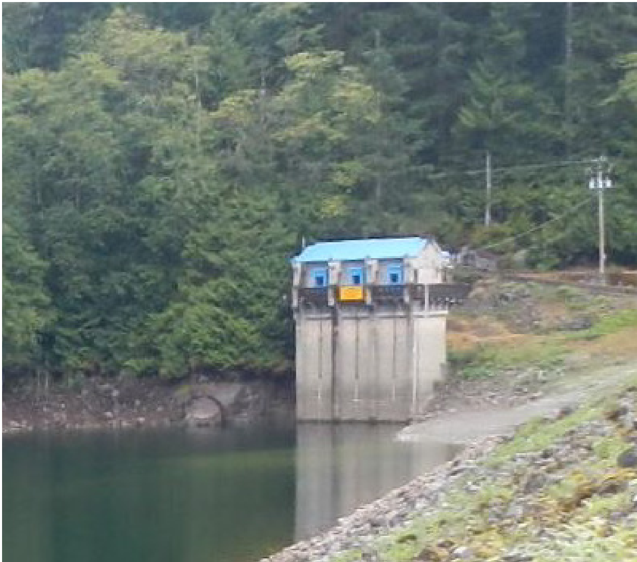
Figure 8. Photograph of Sluice Tower Outlet.
