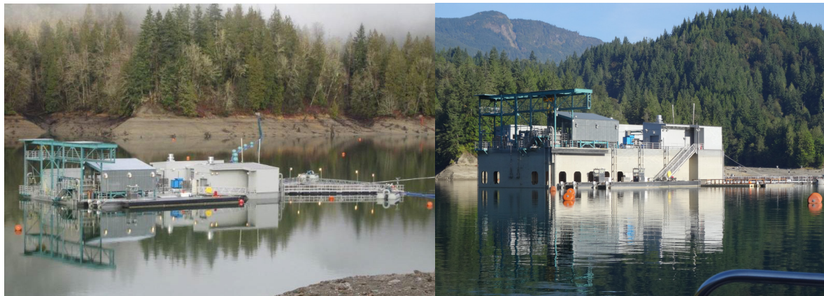
Figure 23. Lower Baker FSC in Operating Position (left) and Raised Non-Operating Position (right).
