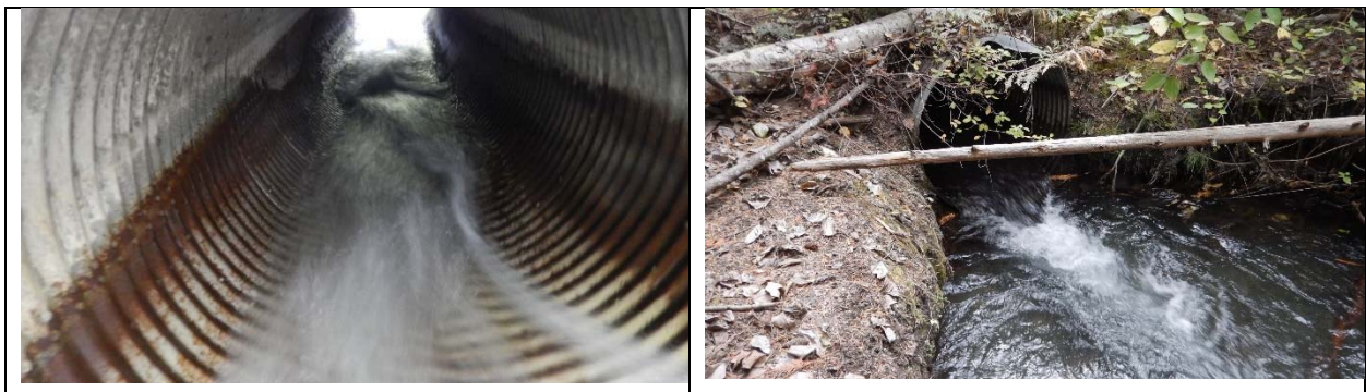
Figure 15. Left- Depth and velocity conditions inside the driveway crossing of Blackwater Creek were characterized by sheet flow conditions, which did not meet criteria for fish passage. Right- The outfall of the driveway crossing of Blackwater Creek was indicative of the high culvert velocity which did not meet criteria for fish passage
