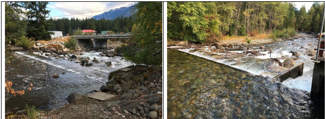
Figure 22. Left: Downstream view of riffle constructed to direct adult Sockeye into the spawning channel. Note sheet flow conditions at the upstream control weir, as well as hydraulic jumps, and increased velocity through the riffle. Right: Downstream view of riffle constructed as part of the spawning channel intake. Note hydraulic jumps, and increased velocity created by the riffle, and the concrete fish ladder along the right margin.
