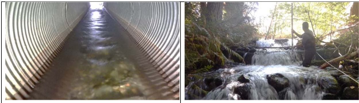
Figure 11. Left: Observed depth and velocity conditions inside the Portage Road crossing of Blackwater Creek appeared to meet criteria for fish passage. Right: Drop heights, and pool depth to jump height ratios associated with weirs downstream of the Portage Road crossing of Blackwater Creek did not meet criteria for fish passage.
