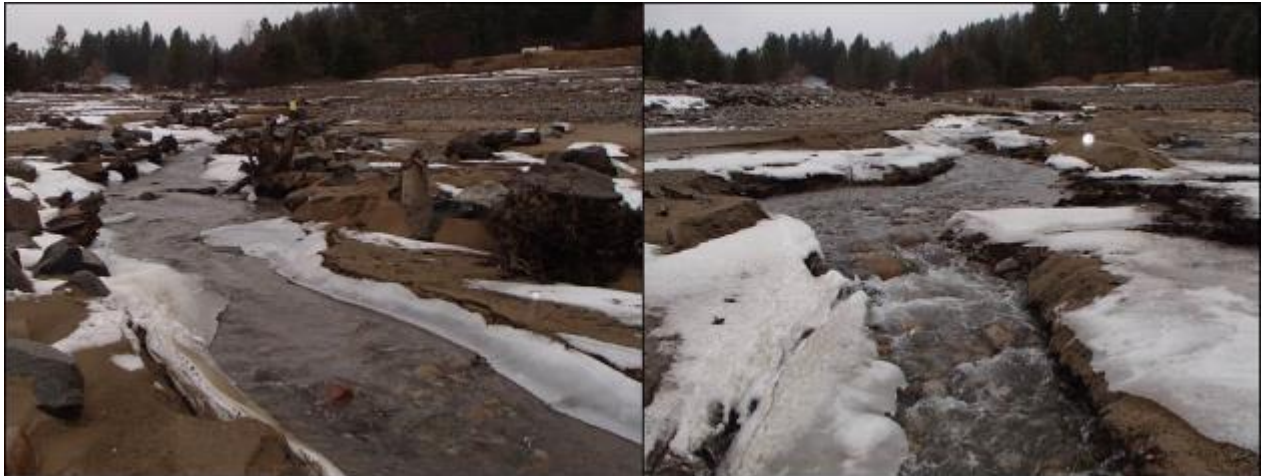
Figure 36. (Left) Phase II Habitat structures, from a downstream perspective, forming banks in the drawdown zone contributing to the formation of a single defined channel; (right) Deer Creek in a defined channel flowing through the drawdown zone downstream of Phase I & II structures from a downstream perspective. Photos by Evan Smith, Okanagan Nation Alliance, March 2018.
