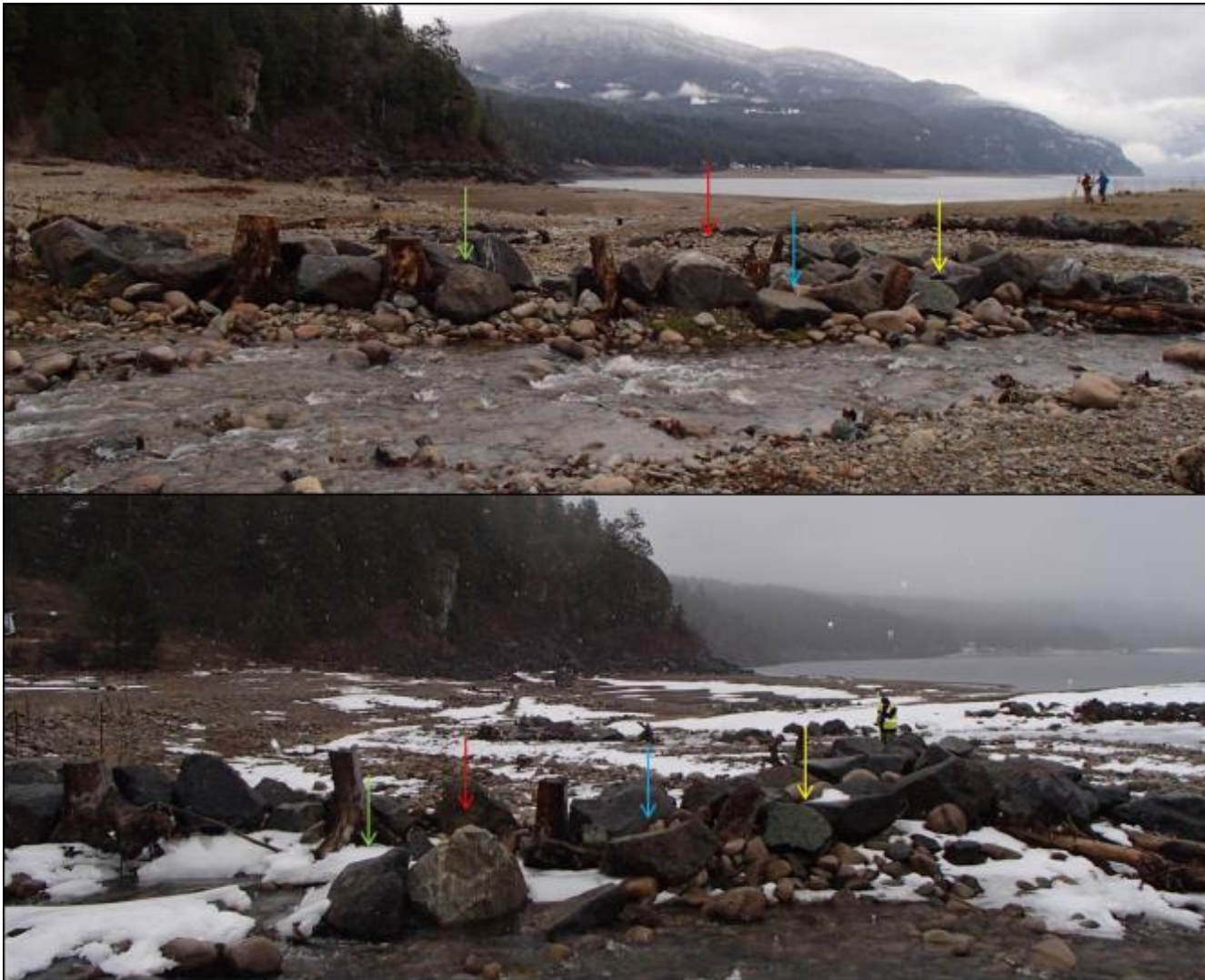
Figure 23.(Top) Structure 5 post -construction in November 2015 with coloured arrows (green, red, blue, yellow) highlighting the positions of four specific rocks; (bottom) Structure 5 in March 2018 after two years of being subjected to freshet and reservoir inundation with coloured arrows (green, red, blue, yellow) highlighting the movements of specific rocks. Photos by Evan Smith, Okanagan Nation Alliance, November 2015 and March 2018).
