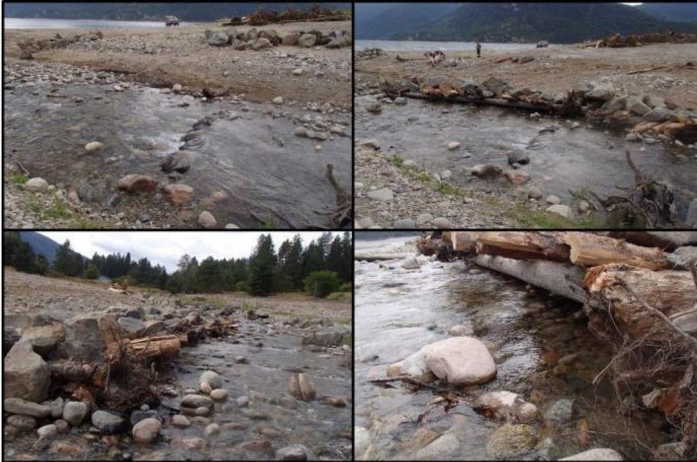
Figure 7. Before (top left) and after (top right) comparison from a upstream perspective of Structure 9 on the right bank in the section of Deer Creek within the drawdown zone; (bottom left) closer view of Structure 9 from a downstream perspective depicting overhanging cover for Kokanee; (bottom right) Close up of the artificial cut banks that fish can utilize for cover. Photos by Evan Smith, Okanagan Nation Alliance, August 2016.
