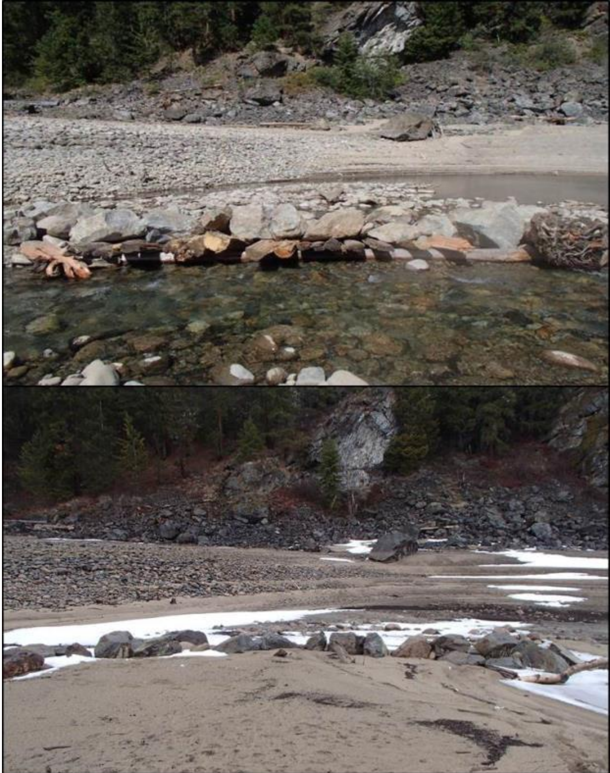
Figure 33. (Top) Structure 19 post -construction in August 2016; (bottom) Structure 17 in March 2018 after one year of being subjected to freshet and reservoir inundation. Photos by Evan Smith, Okanagan Nation Alliance, August 2016 and March 2018).
