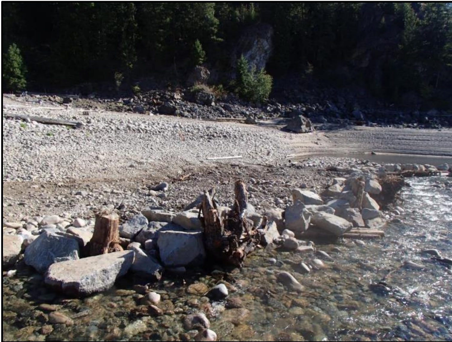
Figure 46. Structure 16 post-construction from an upstream perspective on August 12 th 2016. Photo by Evan Smith, Okanagan Nation Alliance, August 2016..
