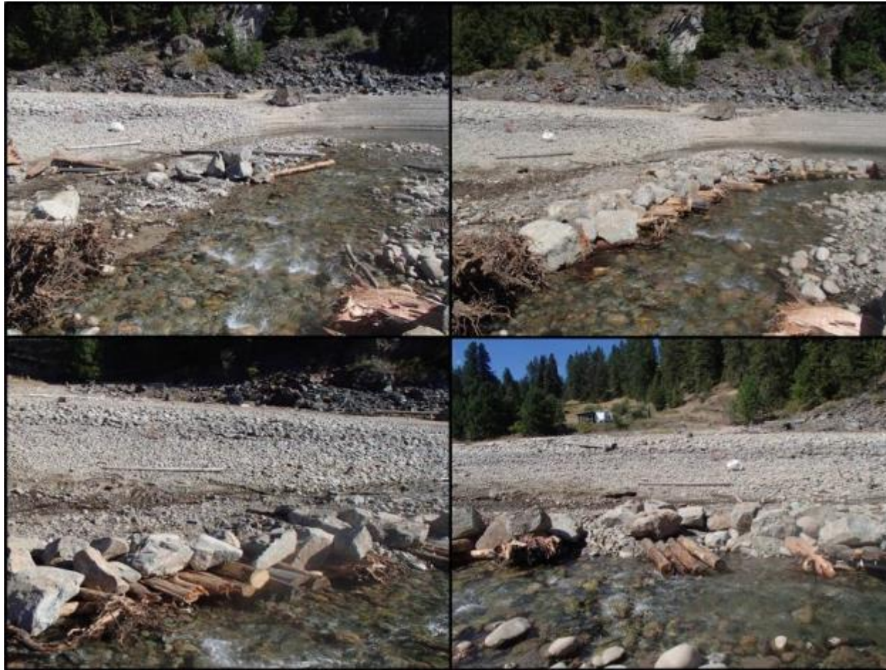
Figure 15. Before (top left) and after (top right) comparison of Structure 18 from an upstream perspective on the left bank in the Deer Creek drawdown zone; (bottom left) closer view of Structure 18 shows its use as cover; (bottom right) four logs at the end of Structure 18 that are designed to create a pool for Kokanee refuge based on monitoring results of Structure 8 in Phase I. Photos by Evan Smith, Okanagan Nation Alliance, August 2016.
