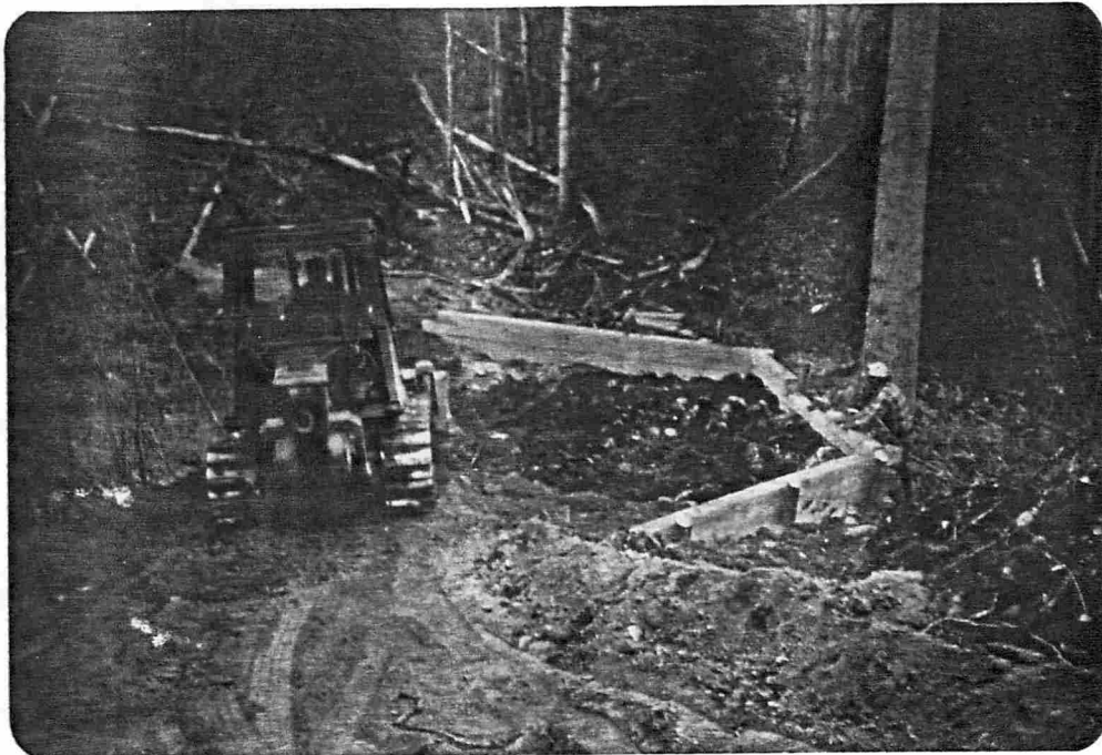
Photo 3. Back-filling the crib-outlet stream fish barrier.
