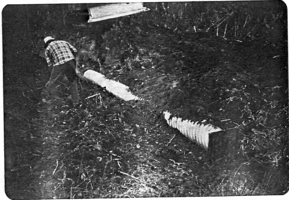
Photo 4. Fish barrier-inlet stream. A screened culvert has been placed into the drainage ditch connecting Vallee Creek to Dunalter Lake.
