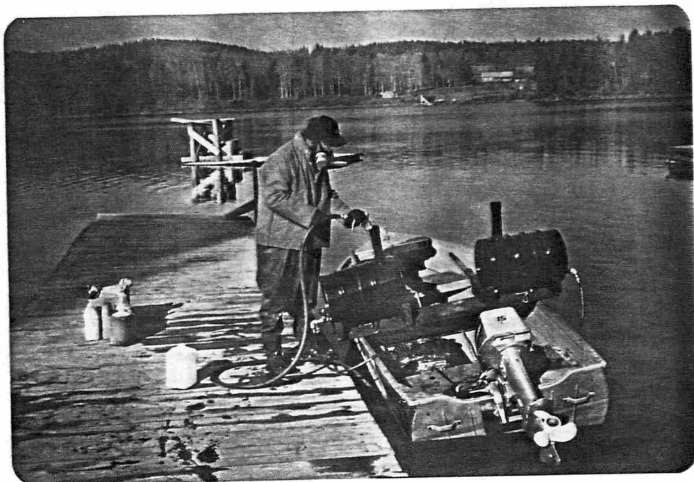
Photo 7. One of the cartop boats, showing the cradles and drums set-up.
