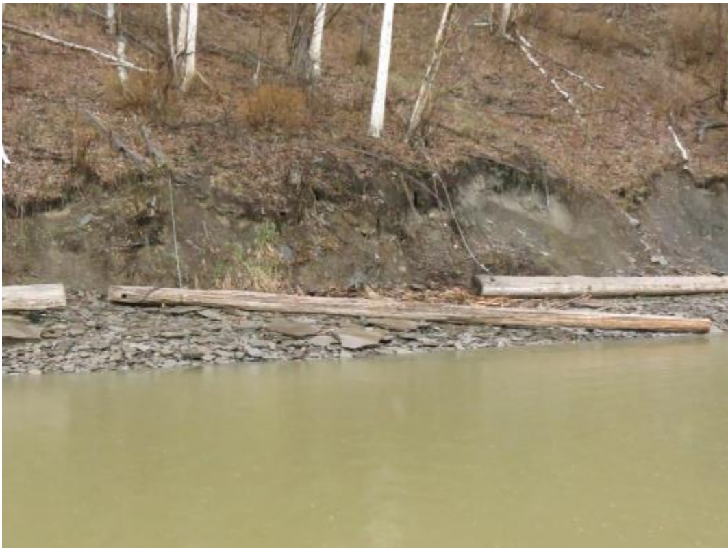
Site 2b and 2c: single anchors but can be a boat hazard at higher water levels.
