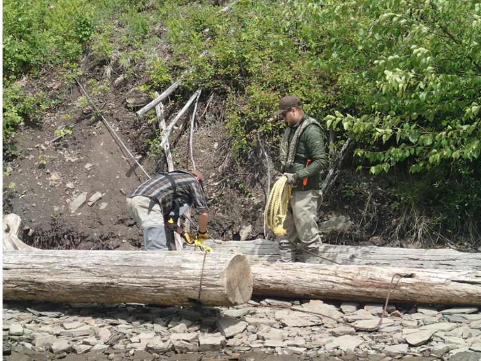
Site 1: An example on how cables are broken and structures are to be secured to the earth anchor again.
