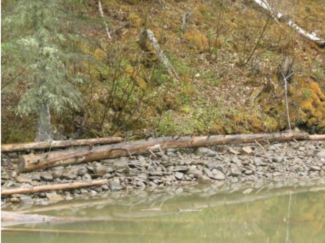
Site 3j2 triangle: note right anchor is tied to a stump, may come loose after a year
