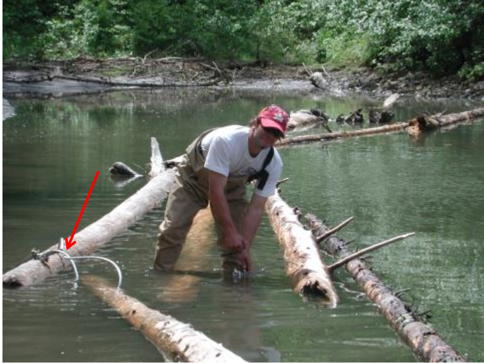
Figure 5. Holes were first drilled in the log and attached together with cables and clamps.
