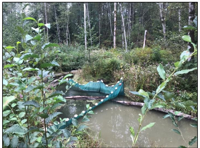
Delivery of boulders, gravel and LWD commences, erosion and sediment control installed
