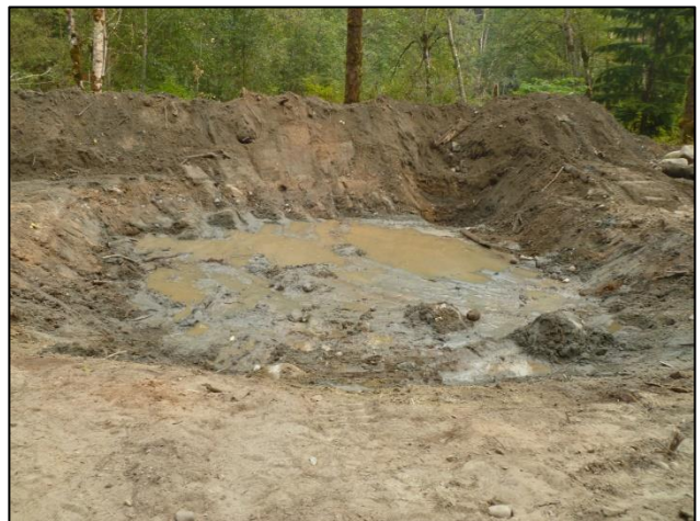
Sediment Detention Pond preparation for water distribution vault before and after
