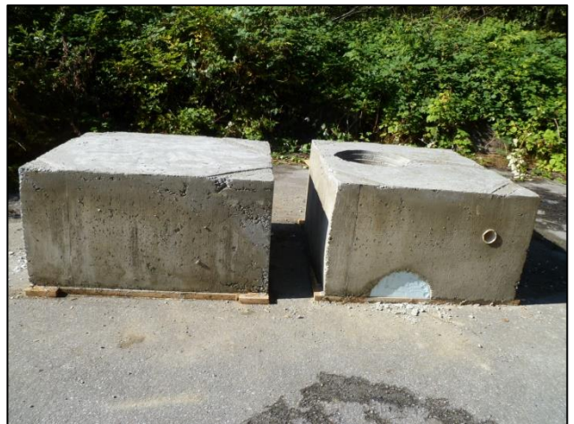
Water distribution vault forms built, cement poured, and forms removed
