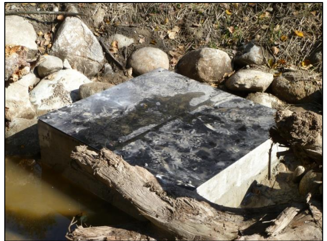
Water distribution vault assembly (top left), embedment into sediment pond (top right) river water connection pipe assembly (bottom left), steel lid installation (bottom right)
