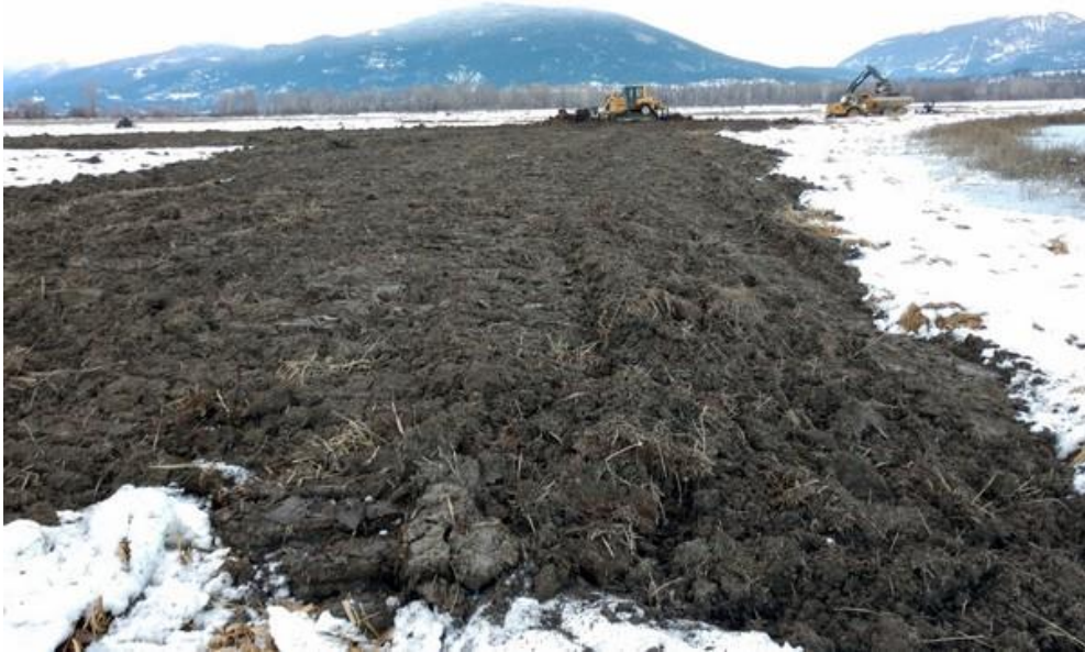
Soil removed from building wetlands was shaped into naturally appearing uplands.
