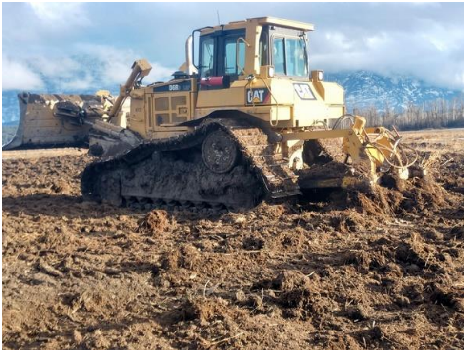
The ripper attachment on the dozer was used to loosen compacted soils over large areas.
