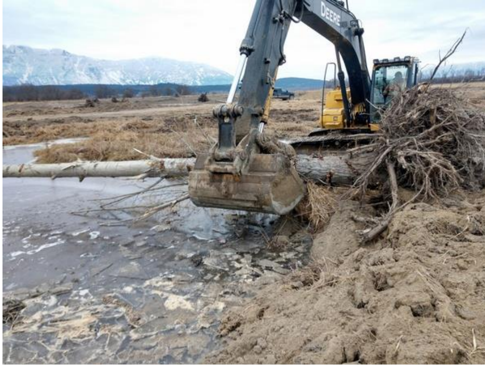
The excavator places large woody debris in a restored wetland to provide the Western painted turtle with basking sites, and waterfowl with loafing sites.
