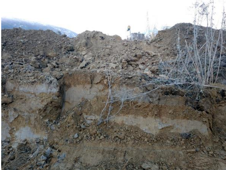
A cross-section dug in the dam surrounding the KUPI Marsh Impoundment. Photos shows where the dam has been built from sand.
