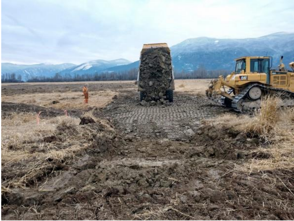
The dump truck and dozer build a core trench across a ditch to restore Wetland 3.
