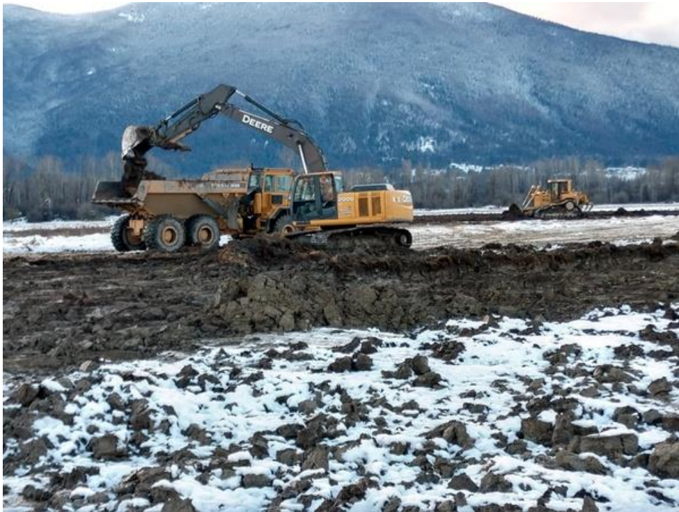
An excavator, off-road dump truck, and dozer were used to restore wetlands.
