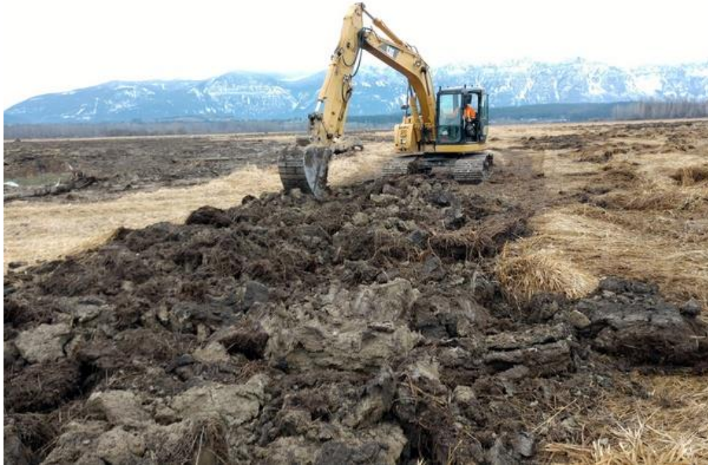
The excavator was also used to loosen soils compacted by the dump truck.
