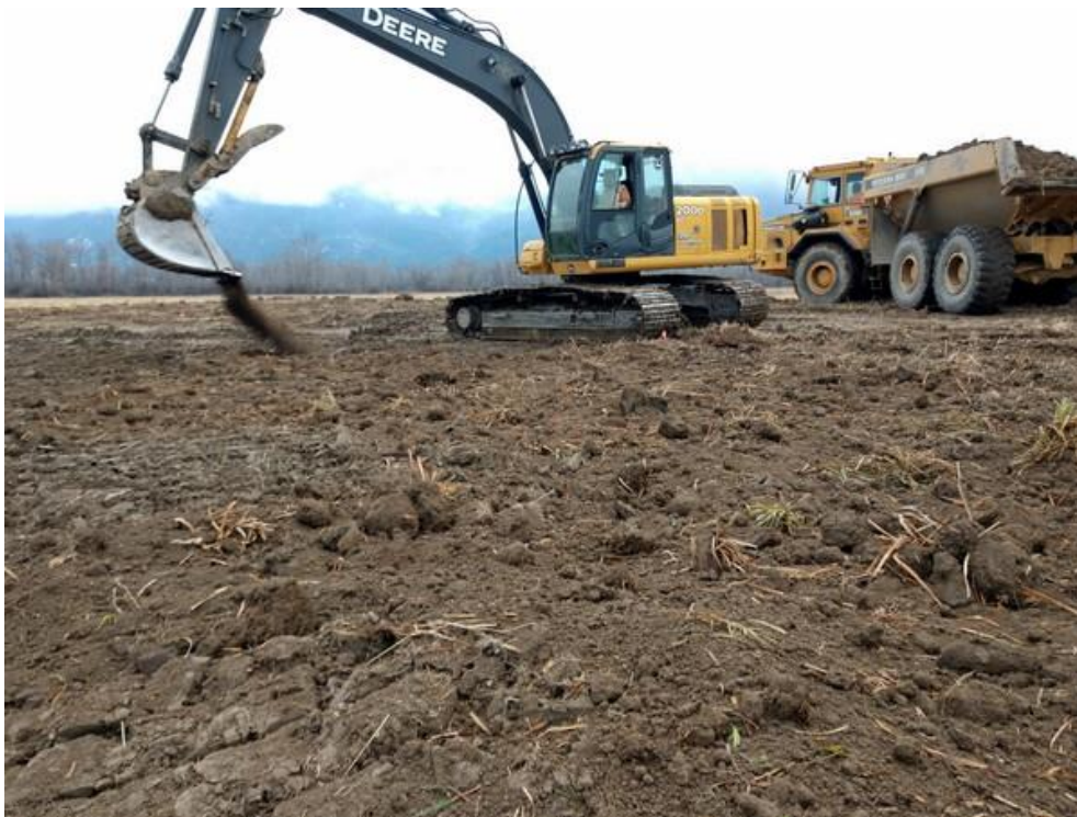
The excavator spreads native sedges around the perimeter of a restored wetland. The dump truck was used to transport the sedges that were salvaged from a ditch that was filled.
