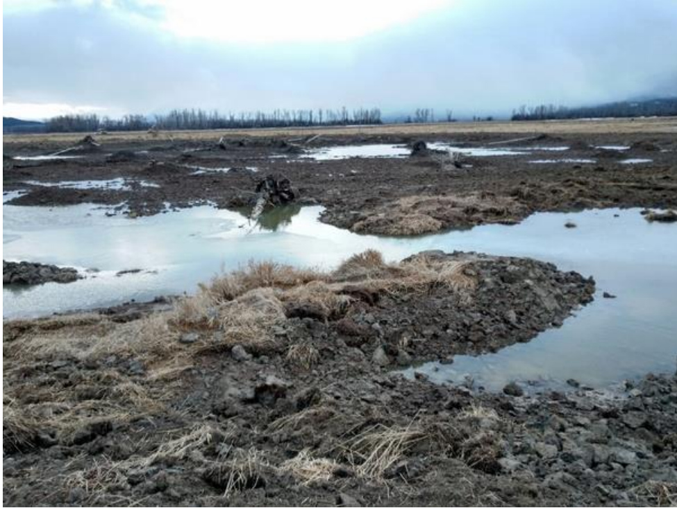
Ditch restored as part of Wetland 1
