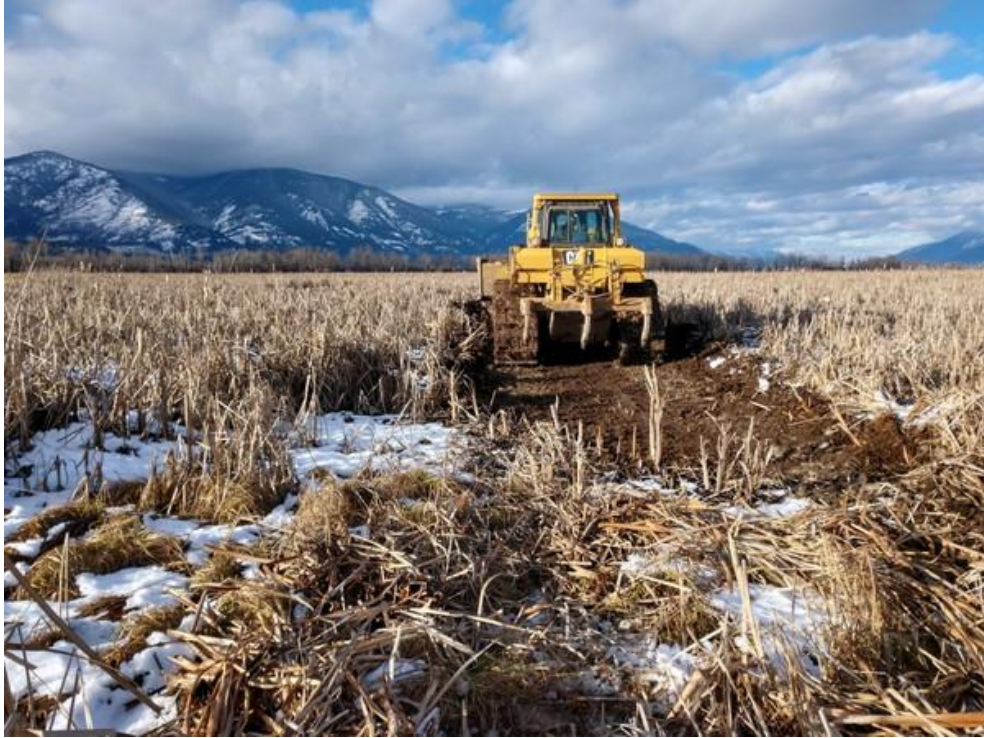
The dozer removes cattails to build a portion of Wetland 6.
