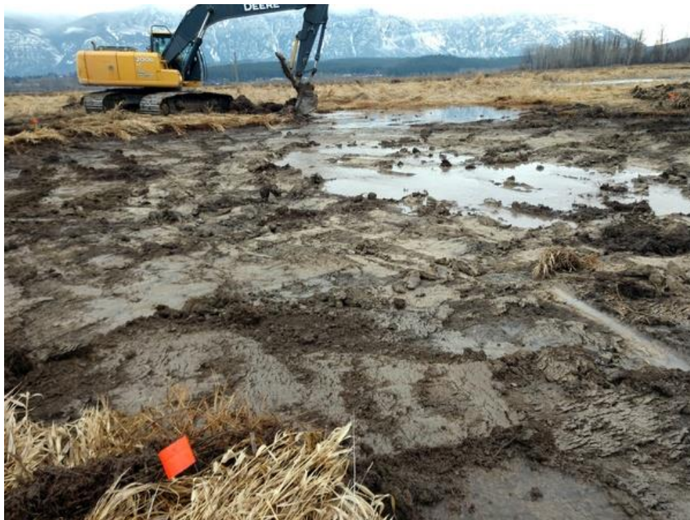
Here Wetland 4 is being shaped by the excavator.
