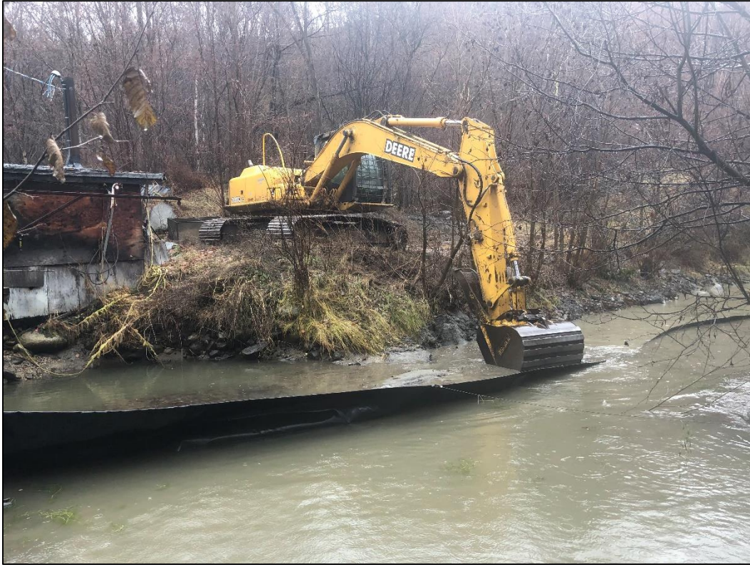
Figure 9: Excavator dredging settling pond.
