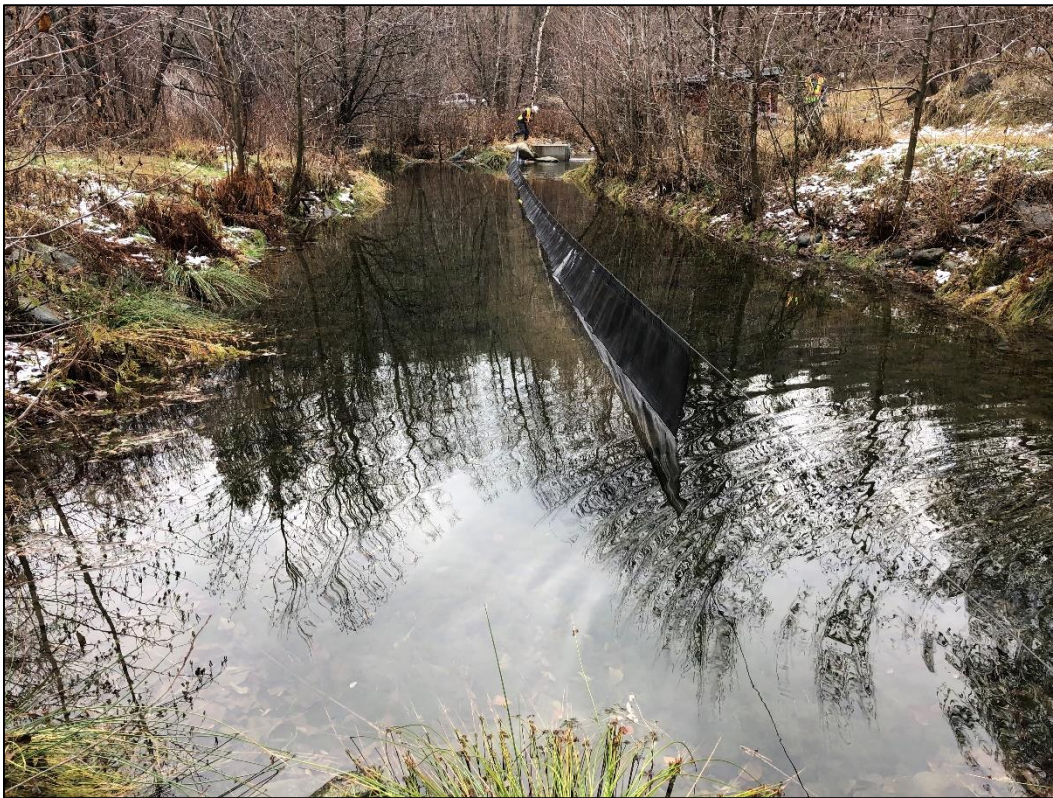
Figure 8: North end of sediment settling pond (looking south) prior to in-water works.
