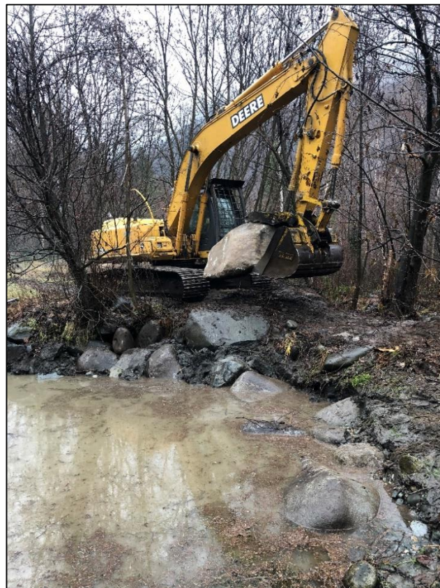
Figure 10: Excavator re-contouring and armoring bank between settling pond and spawning channel.
