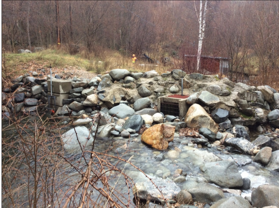
Photo 1. View N of spawning channel intake with Birchbank Golf Course pumphouse in background. Note the boulders surrounding the intake, which have been transported in part by the seasonal flooding of the creek.
