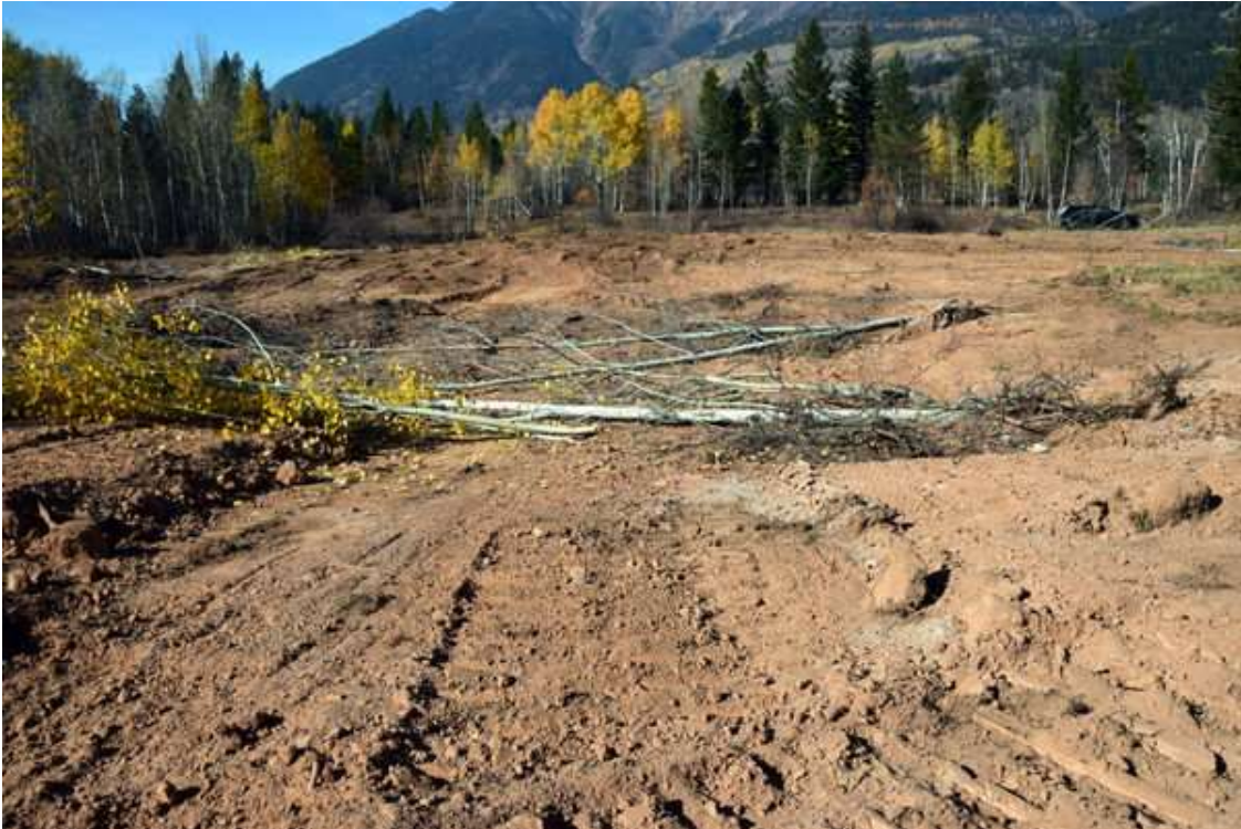
Photo 30: Many of the restored basins are located at the bottom of the creek channel
