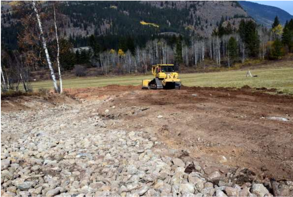
Photo 7: Here a dozer is used to shape a new valley and floodplain for the restored creek along the edge of the existing hayfield.
