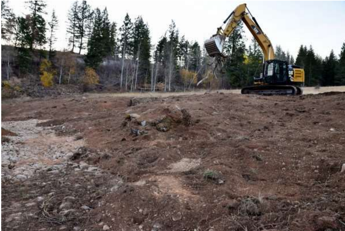
Photo 25: Log, branches, root wads and boulders placed on the restored floodplain to break up homogeneity on the landscape and improve wildlife habitat by providing micro features.
