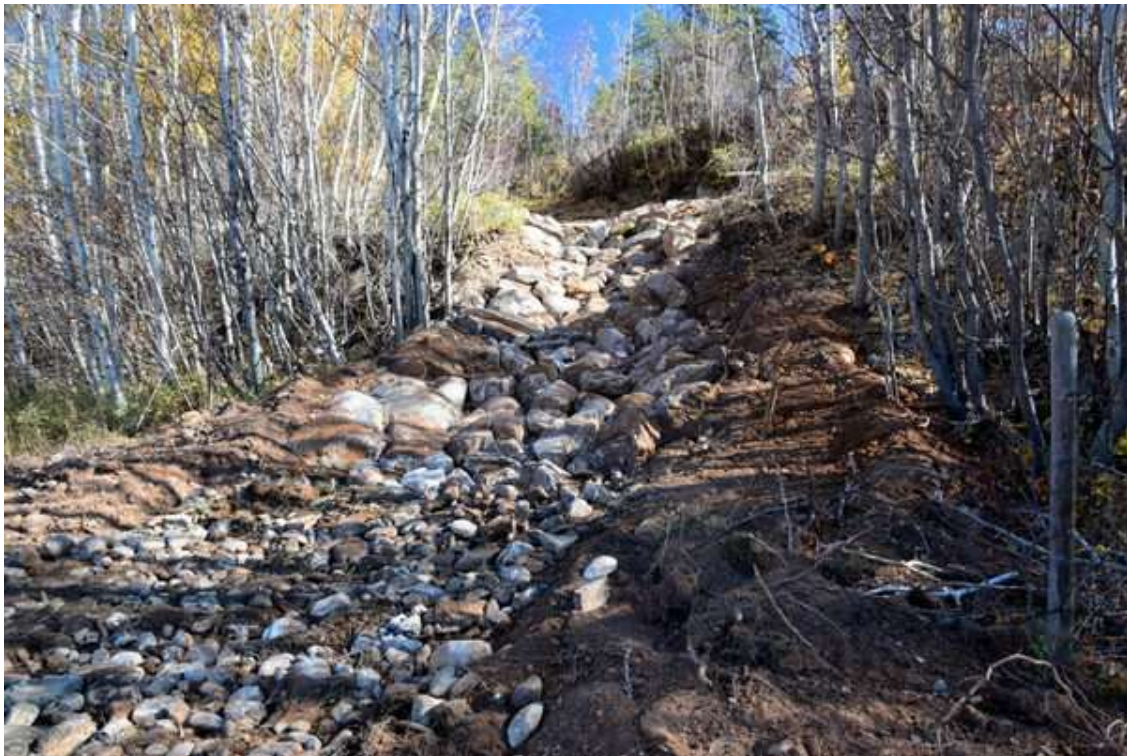
Photo 14: A new valley was restored to replace the flume, moving water from the culvert under the Bull River Forest Service Road into restored Douglas Creek
