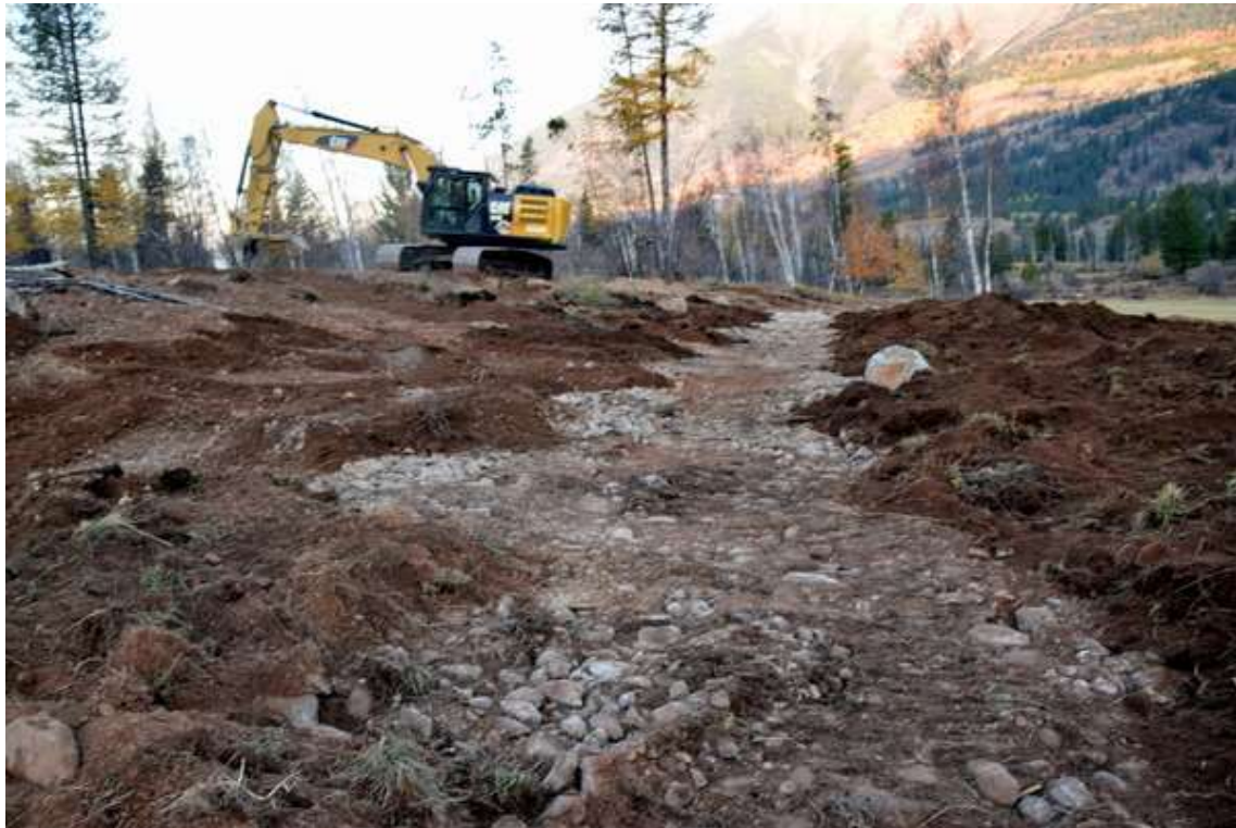
Photo 27: Restored creek and floodplain in progress, looking downslope
