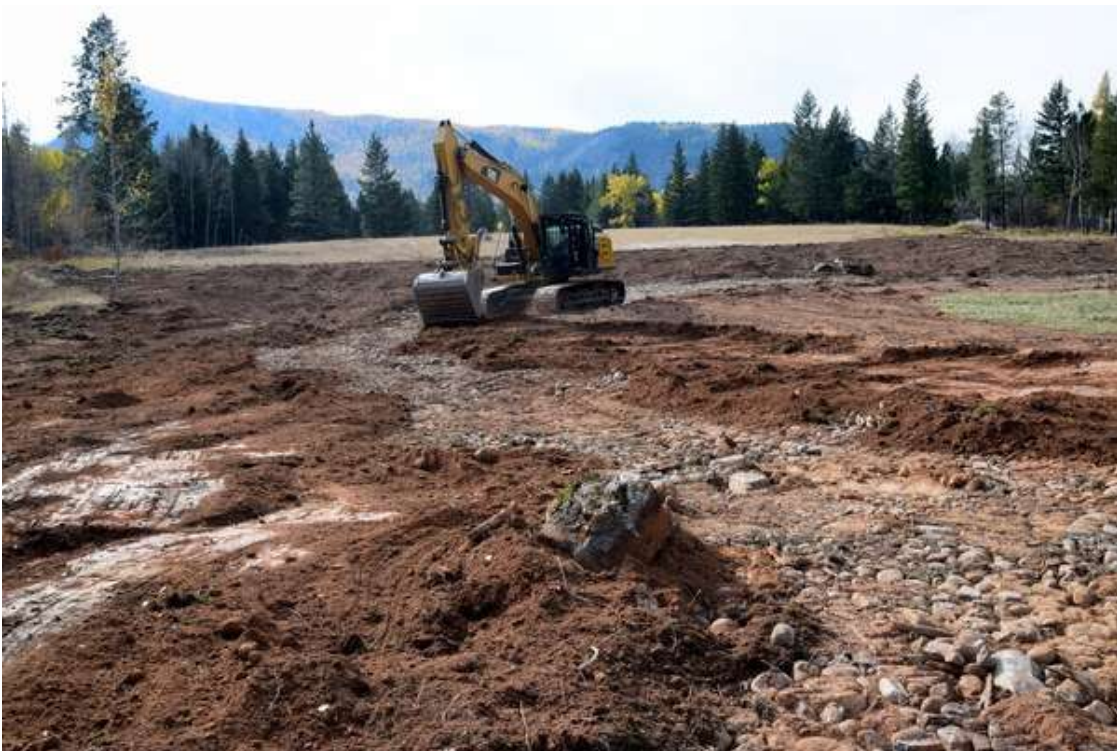
Photo 10: A sinuous floodplain and creek channel are shaped on a gradual slope, in which several wetland basins are designed alongside
