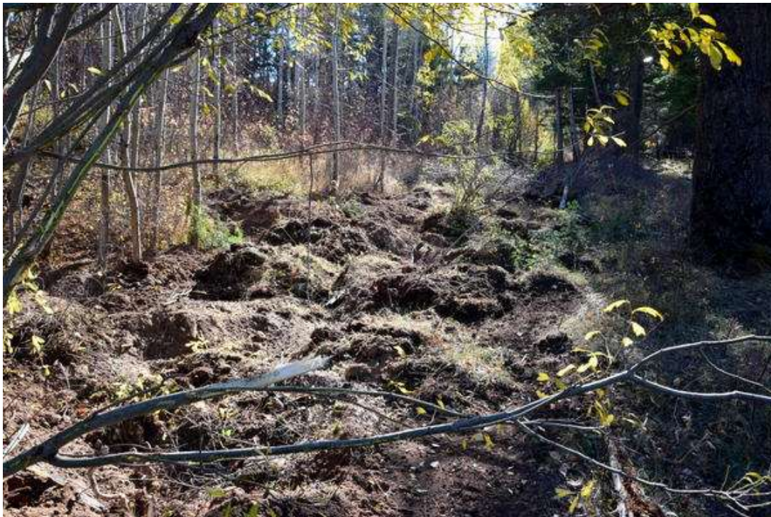
Photo 18: A filled and naturalized section of ditch.
