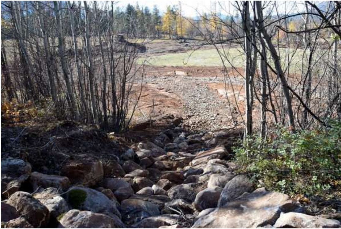
Photo 15: The flume was replaced with a natural rocky valley that would not erode
