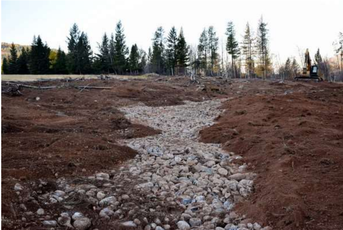
Photo 26: Restored creek and floodplain in progress, looking upslope
