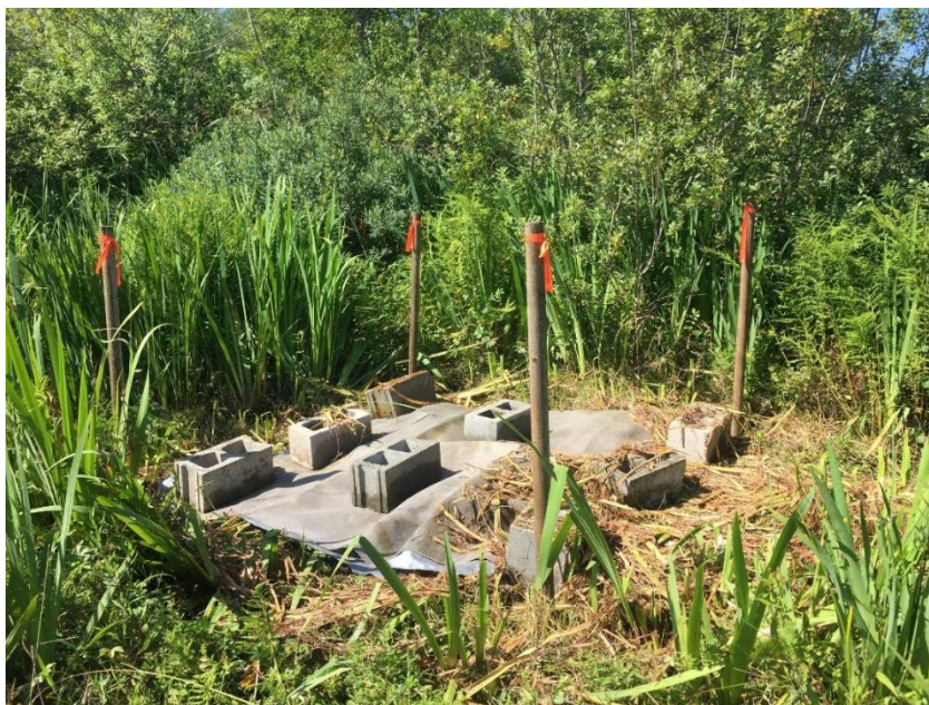
Figure 3: Benthic barrier pilot, July 2018
