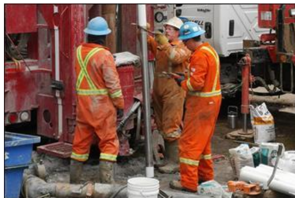
Installation of well screen at Uphill Road.
