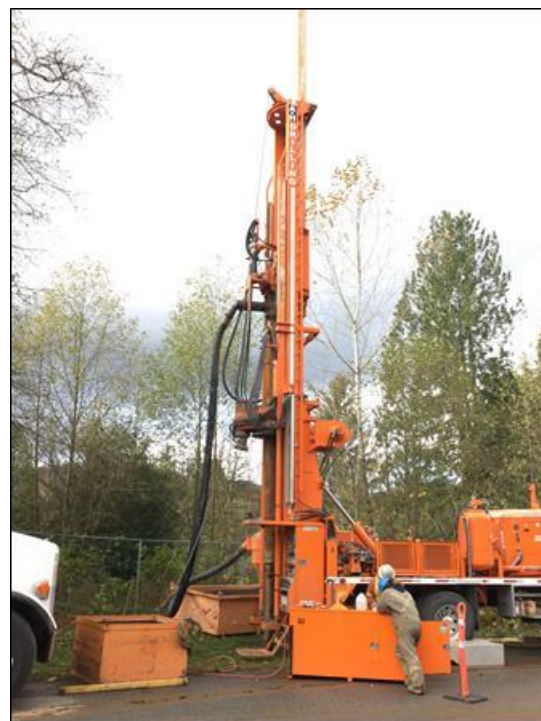
View of dual rotary drill rig at OW479 in Maple Ridge.
