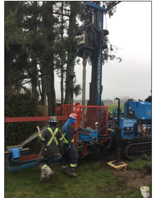
View of sonic drill rig at Observation Well 485 in Dewdney.
