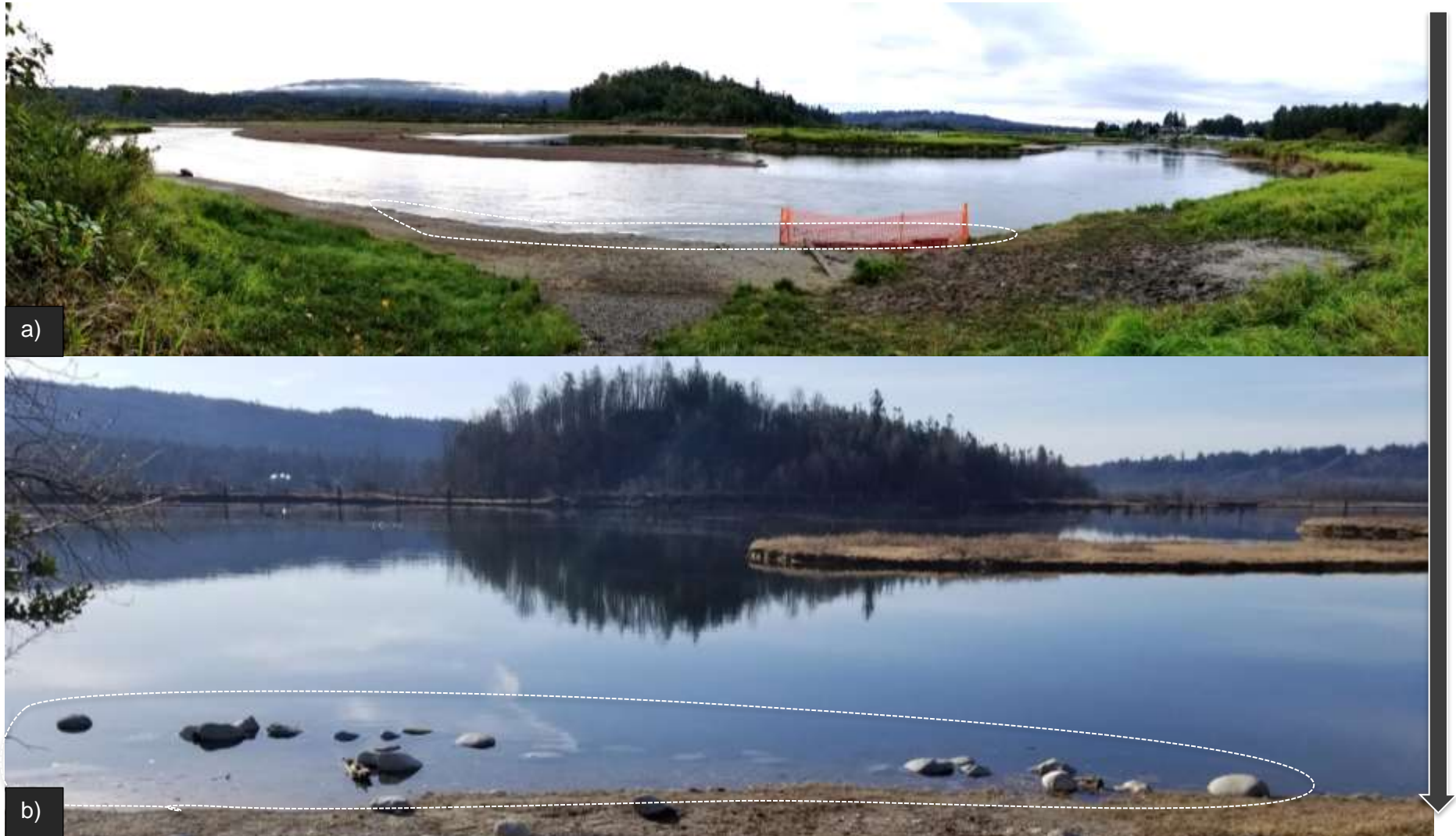
Figure 9. Eastview of the right bank project. a) before reef installed and after excavation of sensitive cultural artifacts. b) After works March 2018 during tail water release. White dashed line delineates reef location.
