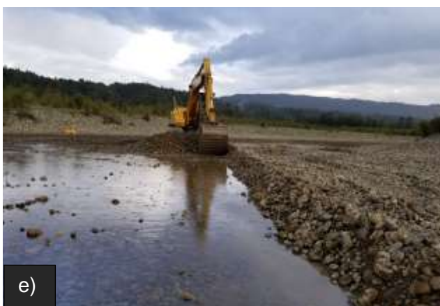
Figure 2. Mainstem rewatering of channel 5. a) excavating berm to create the access path to cross the Stave River. b) Moving gravels to create the access route. c) Excavator safely crosses upstream of Channel 5. d) Re-grading and surveying of gravels begin (notice the dry Channel 5 in proximity to Channel 4). e) east-view illustrating the height of gravel blockage at the upstream end of Channel 5. f) Almost completed Channel 5 watered, needing to push gravels to Channel 4.
