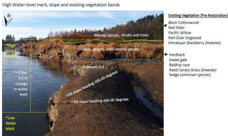
Figure 4. Annotated photo of project site. Notice the erosion of the bank and the lack of existing native trees, shrubs in the riparian. Also notice the presence of invasive reed canary grass. High water mark may be related to higher tail-water flows and freshet levels.
