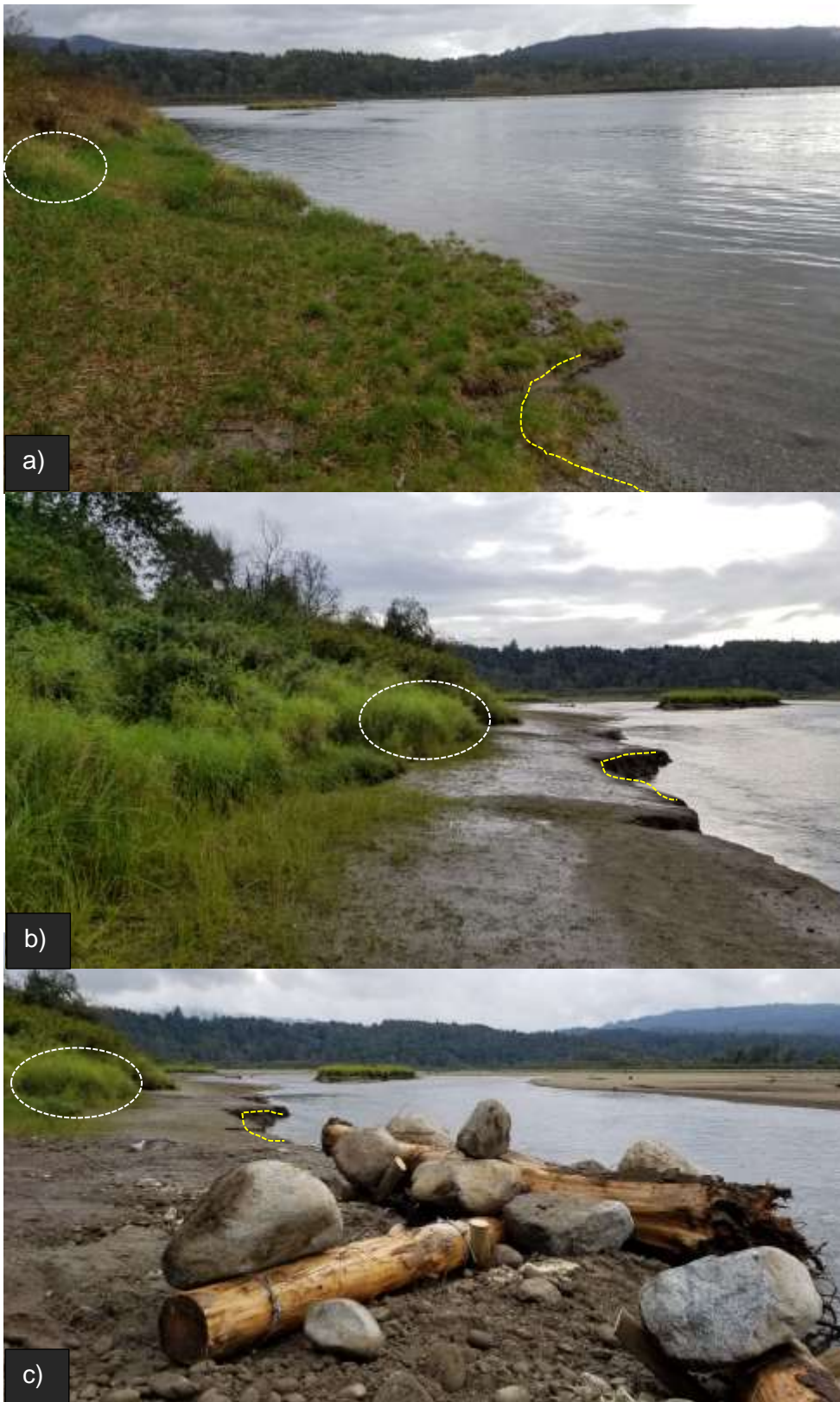
Figure 7. Upstream transition of right bank. a) Before works (May 2018) b) Before works (September 2018) c) after works October 2018. White dashed polygons are location reference points. Yellow dashed lines indicate erosion reference points.
