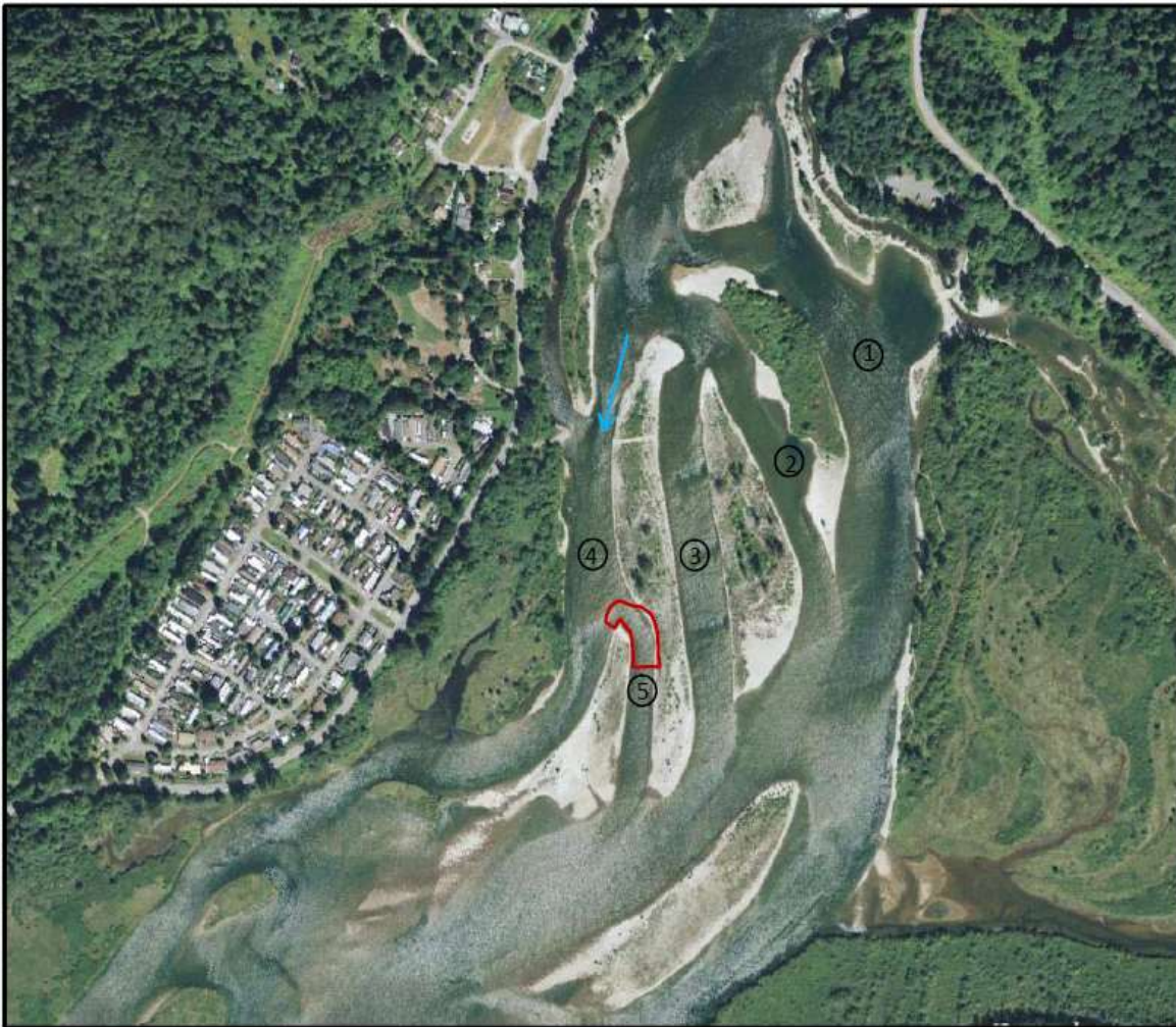
Figure 1. Extracted from Greenback report 2017, red polygon illustrates gravel blockage to channel 5 and significant high-velocity flows down channel 4.
