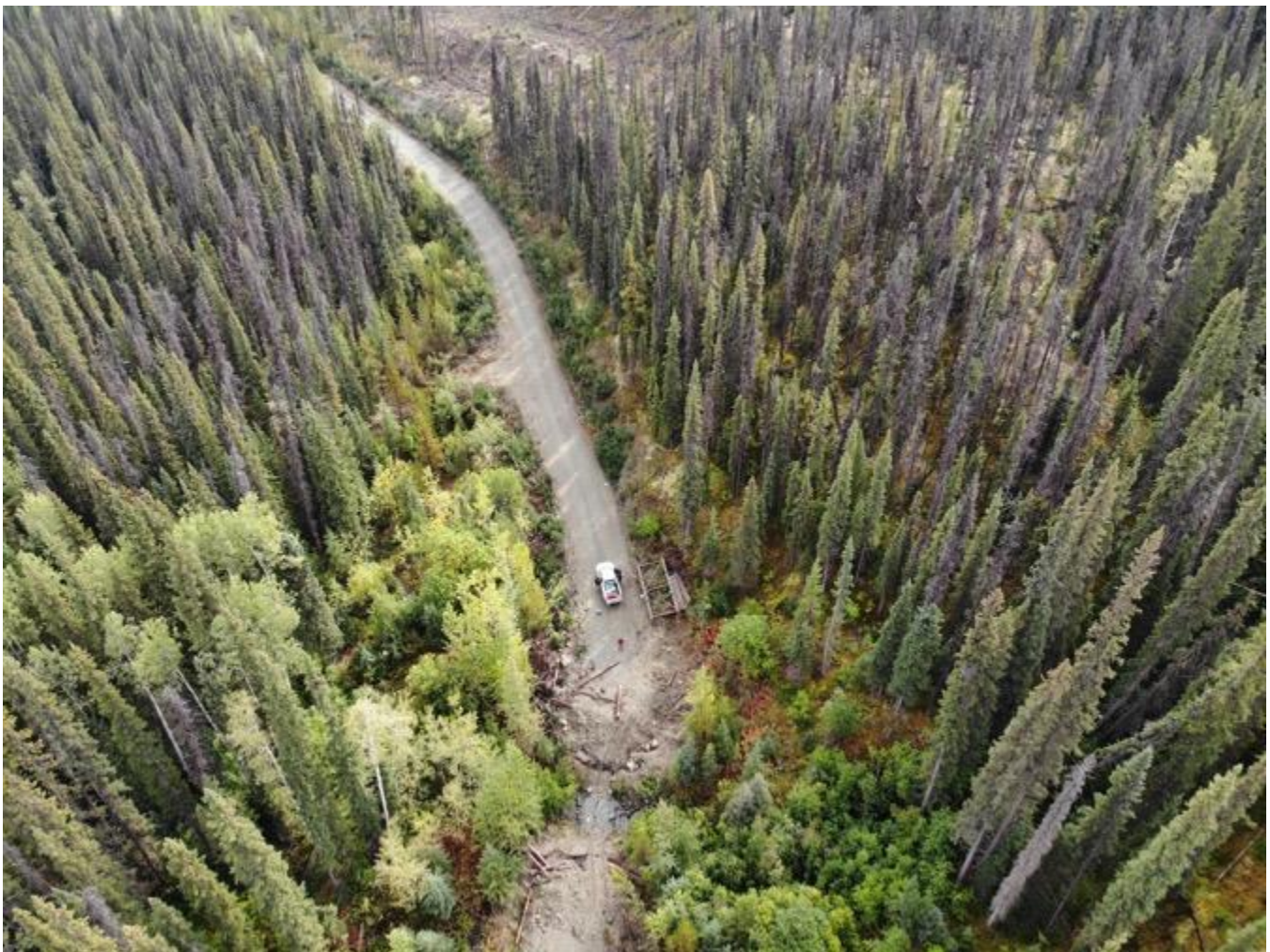
Figure 25. Access control on Tutizzi Lake road (bridge removed).
