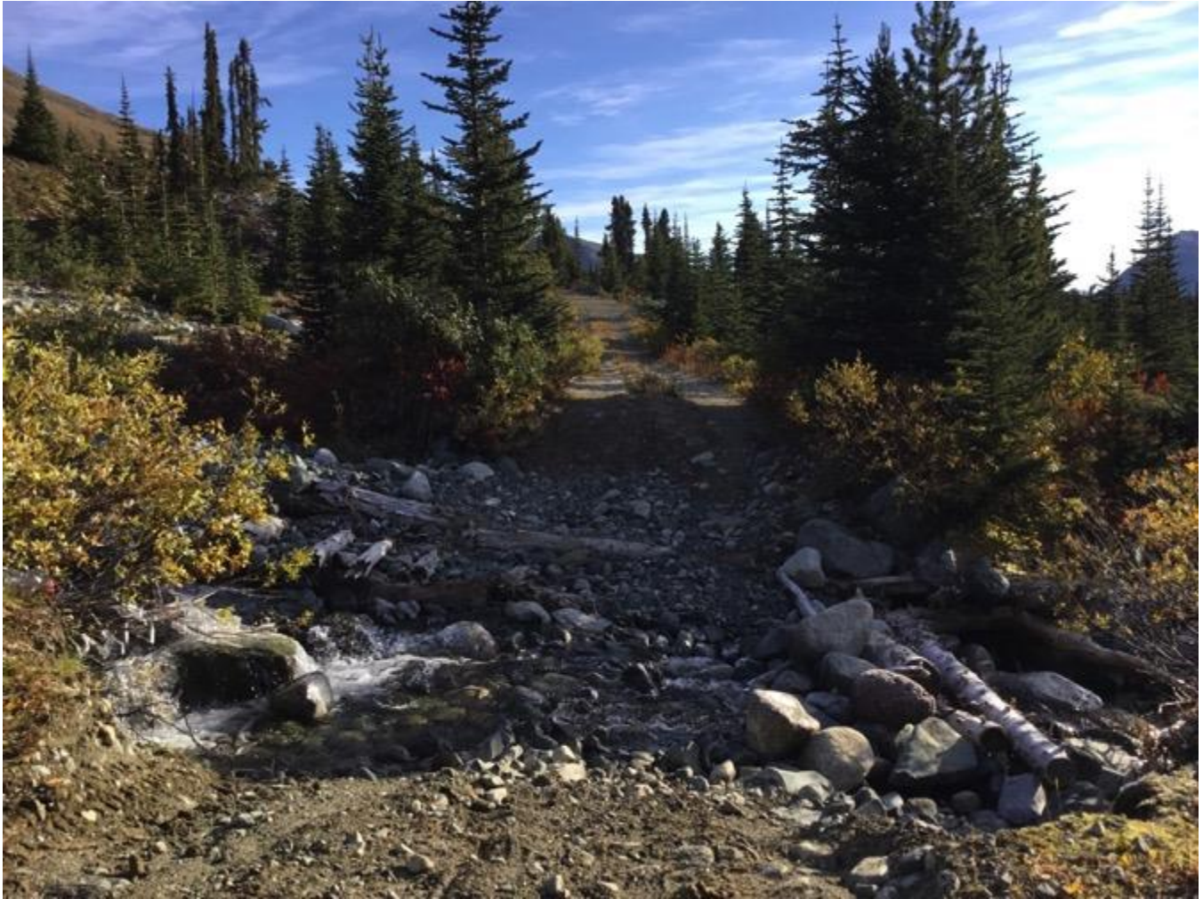
Figure 23. Stream crossing on Road 5.
