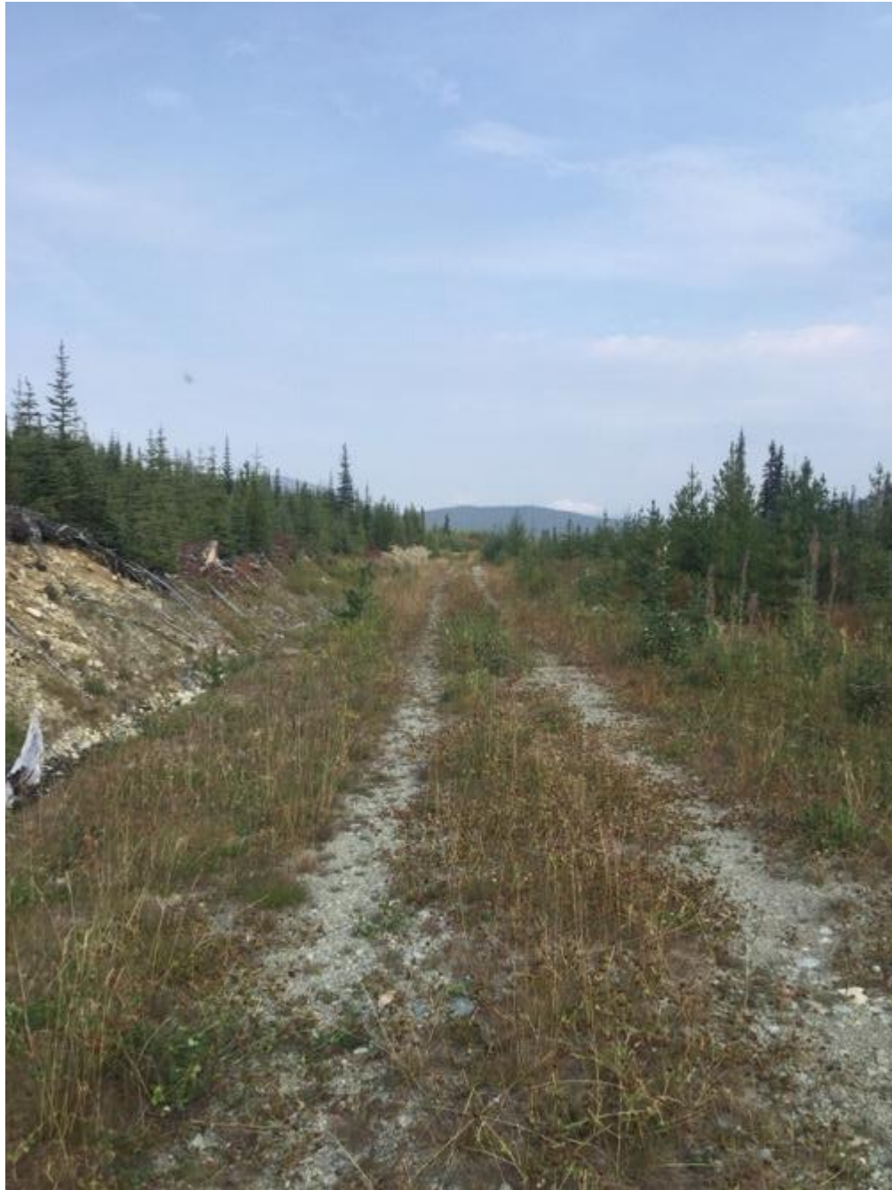
Figure 13. Compaction preventing natural regeneration on Road 1.
