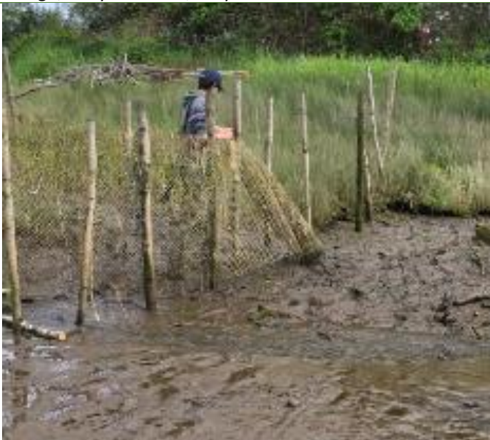
Temporary plastic “snow fencing” coming down to be replaced by 100% natural eco-cultural fencing, constructed of alder, willow, and hemp, May 2019.
