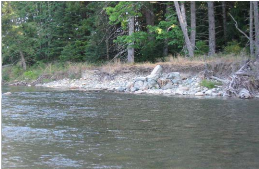
Photo 11. Looking upstream at site 6+140 pre-construction.
