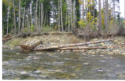
Photo 18. Looking downstream at site 7+180 post-construction.
