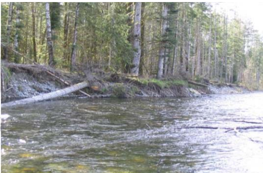
Photo 7. Looking upstream at 5+690 and 5+730 pre-construction.
