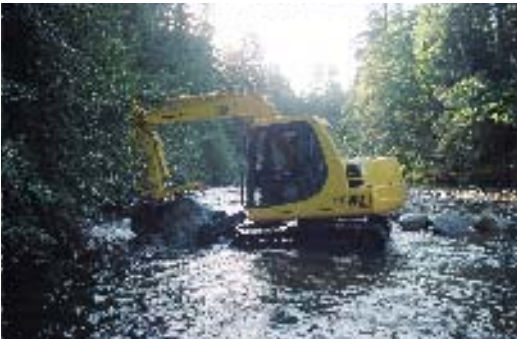
Photo 3. Small excavator placing rocks at riffle site 3+800.
