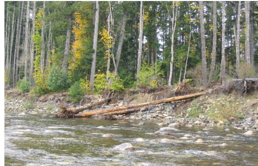
Photo 20. Looking upstream at site 7+220 post-construction.
