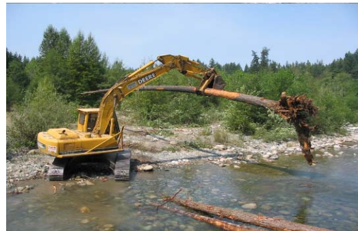
Photo 6. Looking across stream at excavator staging wood at restoration site 6+140.
