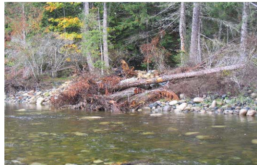
Photo 22. Looking upstream at site 8+805 post-construction.
