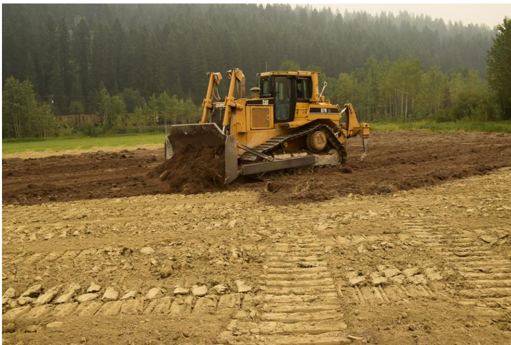
10. Dozer spreading topsoil during restoration at Elk Spike farm
