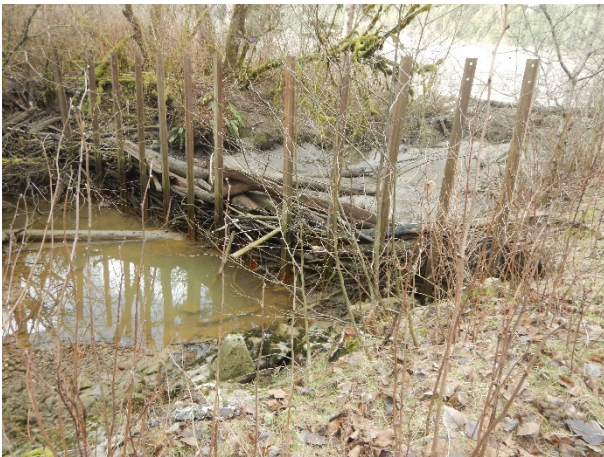
Trash rack at river confluence; note build-up of sediment and woody debris before then after
