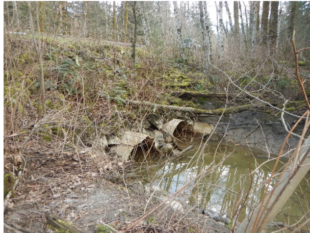
Facing twin culverts from west side of Training Berm (river side): note build up on left photo
