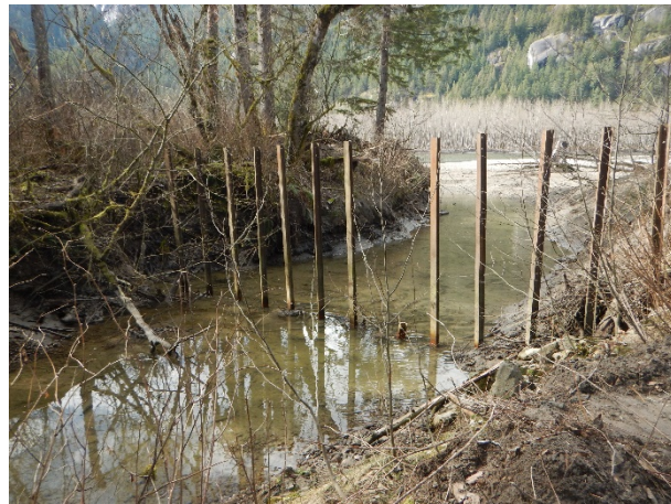
Trash rack at river confluence; note build-up of sediment and woody debris before then after
