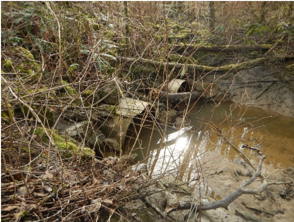
Facing twin culverts from west side of Training Berm (river side): note build up on left photo
