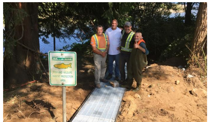
Figure 2. Installed fish ladder with partners and local steward.
