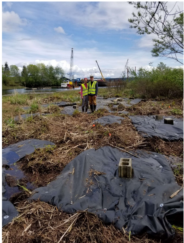
Figure 7: Greenways contractors installing benthic barriers to treat dense areas of yellow flag iris infestation on Baikie Island
