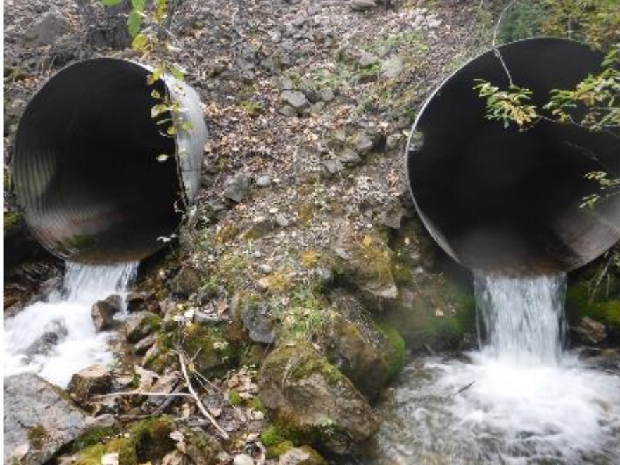
Figure 10: Outlet of PSCIS crossing 57690 (UTM: 10N 555027 6046138).
