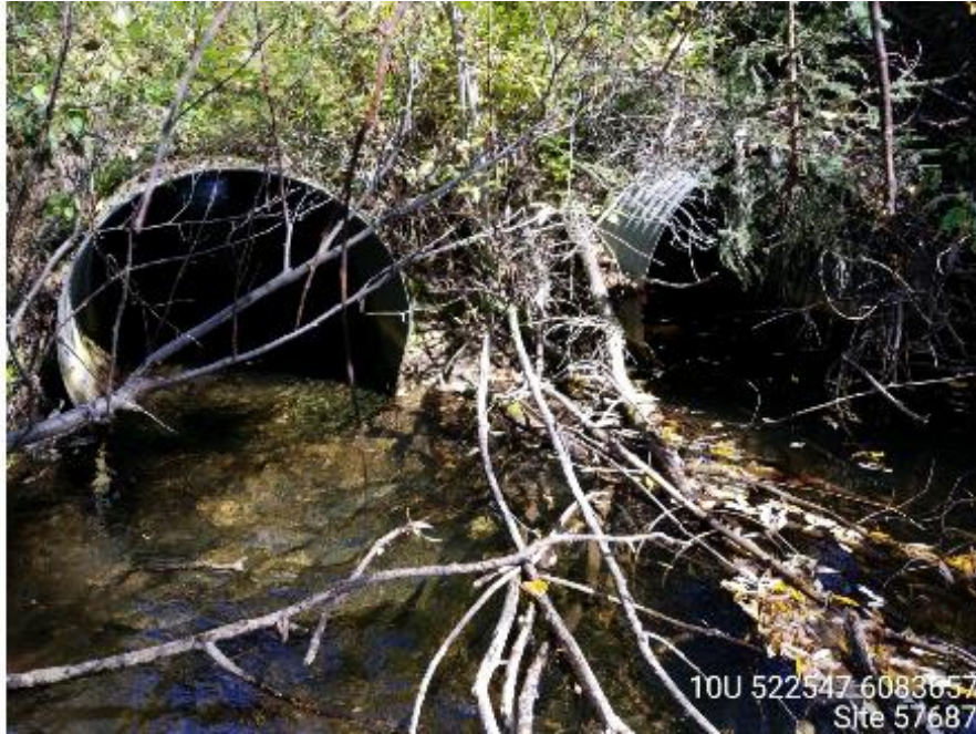
Figure 89: Outlet of PSCIS crossing 125345 (UTM: 10N 522547 6083657).
