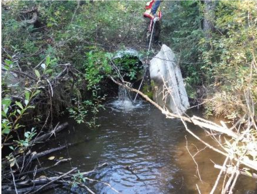
Figure 97: Outlet of PSCIS crossing 125403 (UTM: 10N 520140 6084908).
