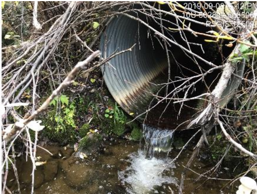
Figure 39: Outlet of PSCIS crossing 125098 (UTM: 10N 582892 6035087).
