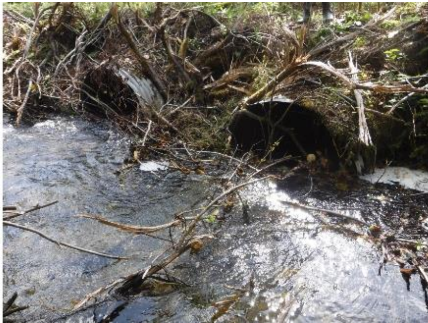
Figure 53: Inlet of PSCIS crossing 125179 (UTM: 10N 570308 6052835).
