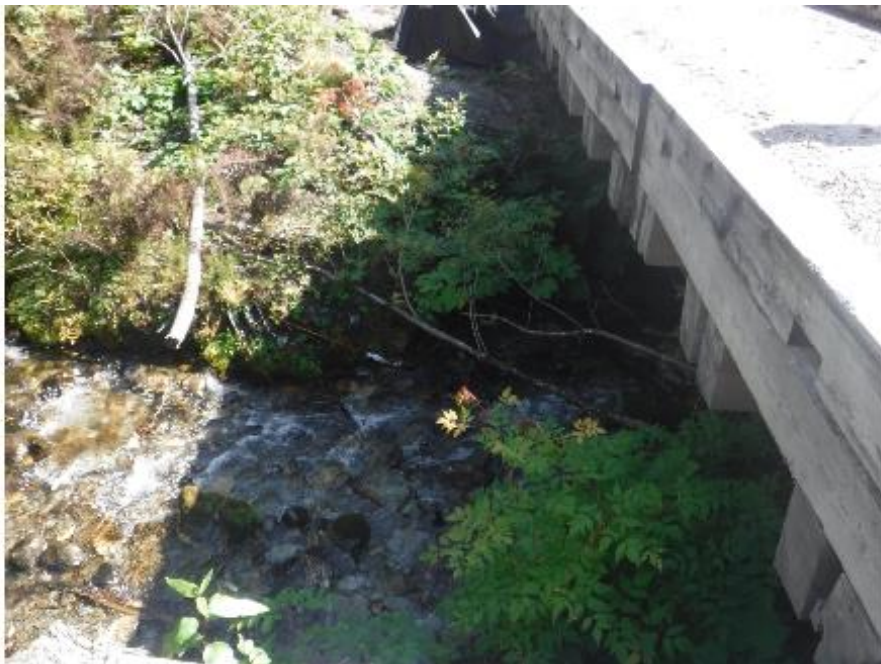
Figure 72: View of bridge (modeled crossing 16603641) located upstream of crossing 125231 (UTM: 10N 550099 6065555).
