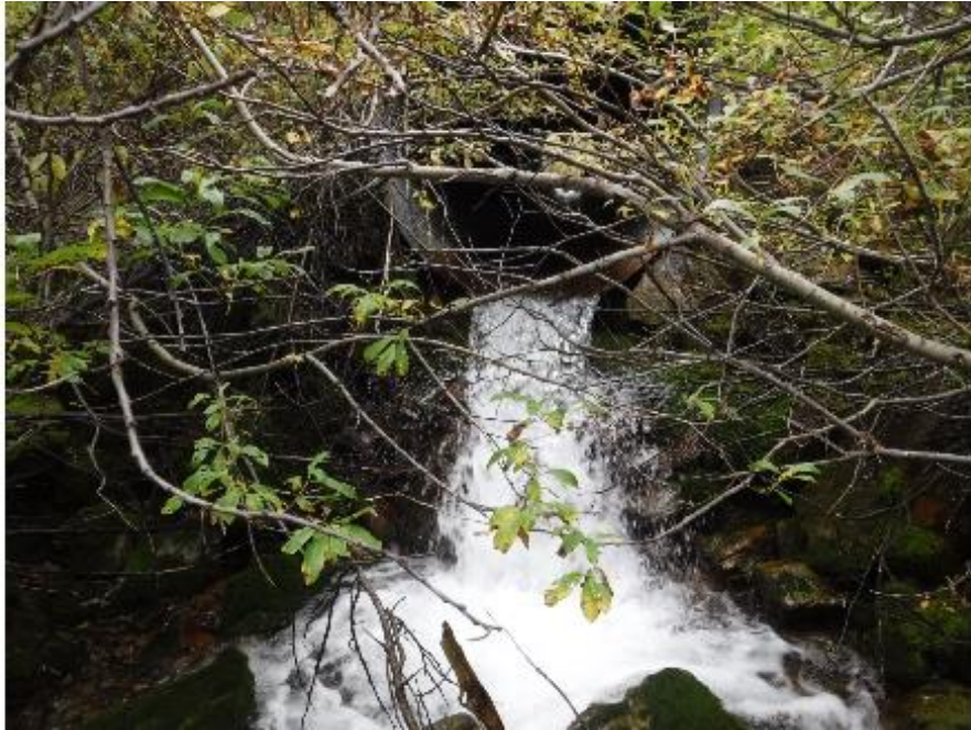
Figure 17: Outlet of PSCIS crossing 57695 (UTM: 10N 563257 6038803).
