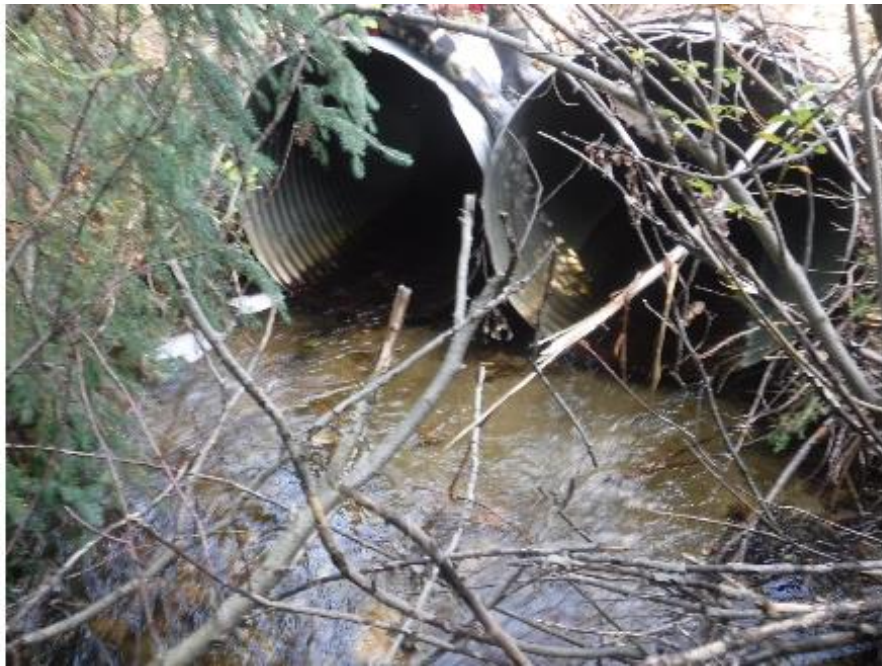
Figure 48: Outlet of PSCIS crossing 125175 (UTM: 10N 571772 6051998).
