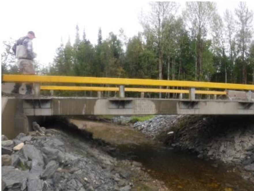
Figure 103: Newly installed bridge located downstream of crossing CV1 (UTM: 10N 547474 6063810).
