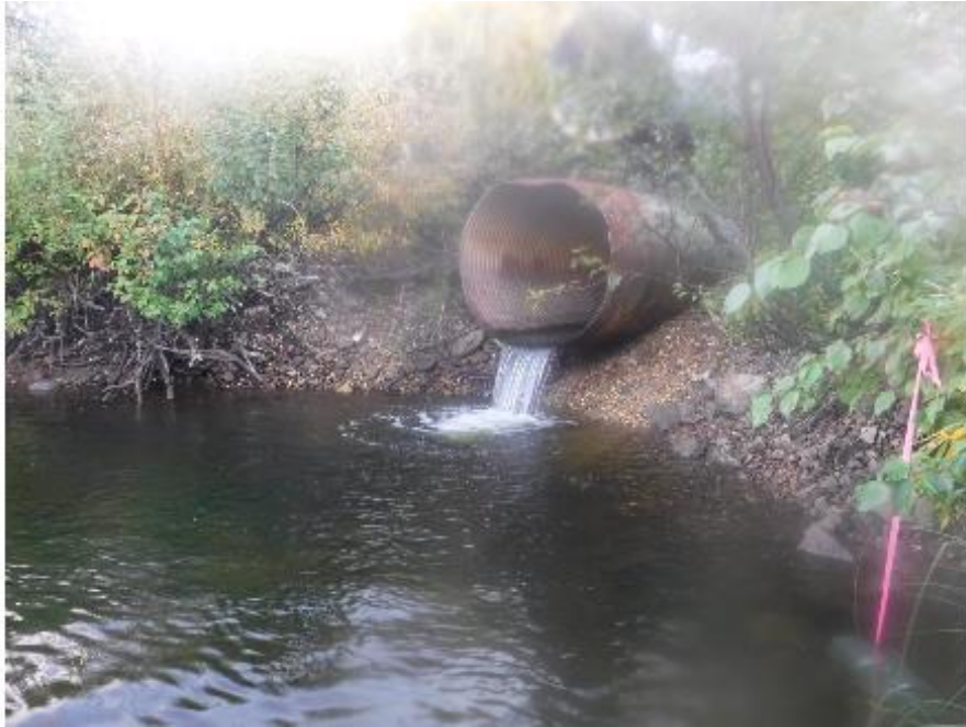
Figure 4: Outlet of PSCIS crossing 57681 (UTM: 10N 533218 6067620).
