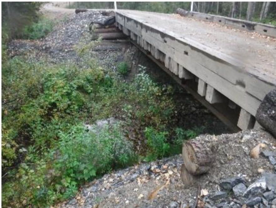
Figure 109: View of bridge located upstream of crossing CV1 (UTM: 10N 549707 6064989).
