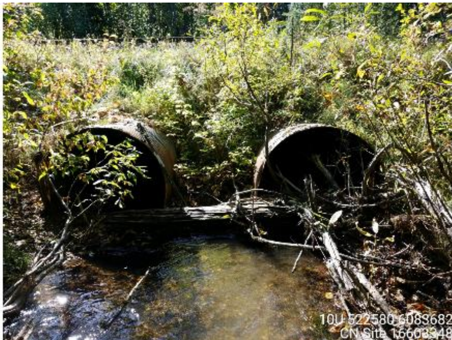
Figure 90: Inlet of PSCIS crossing 57687 (UTM: 10N 522580 6083682).
