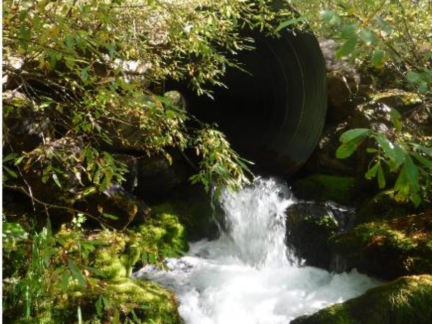
Figure 23: Outlet of PSCIS crossing 57696 (UTM: 10N 564171 6037942).
