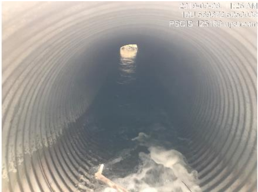
Figure 58: Inlet of PSCIS crossing 125180 (UTM: 10N 569673 6053040).
