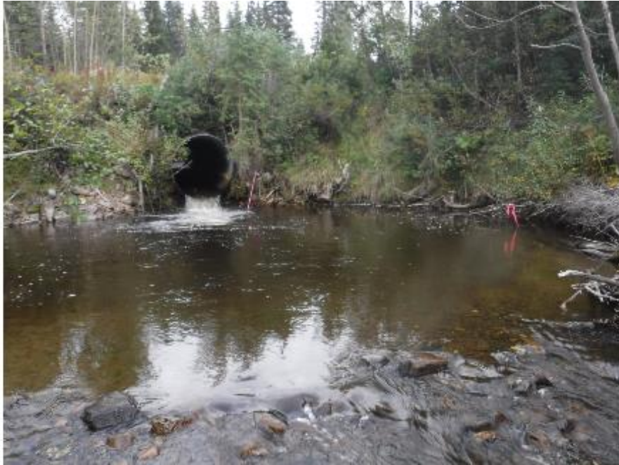
Figure 31: Outlet of PSCIS crossing 125000 (UTM: 10N 577534 6038205).
