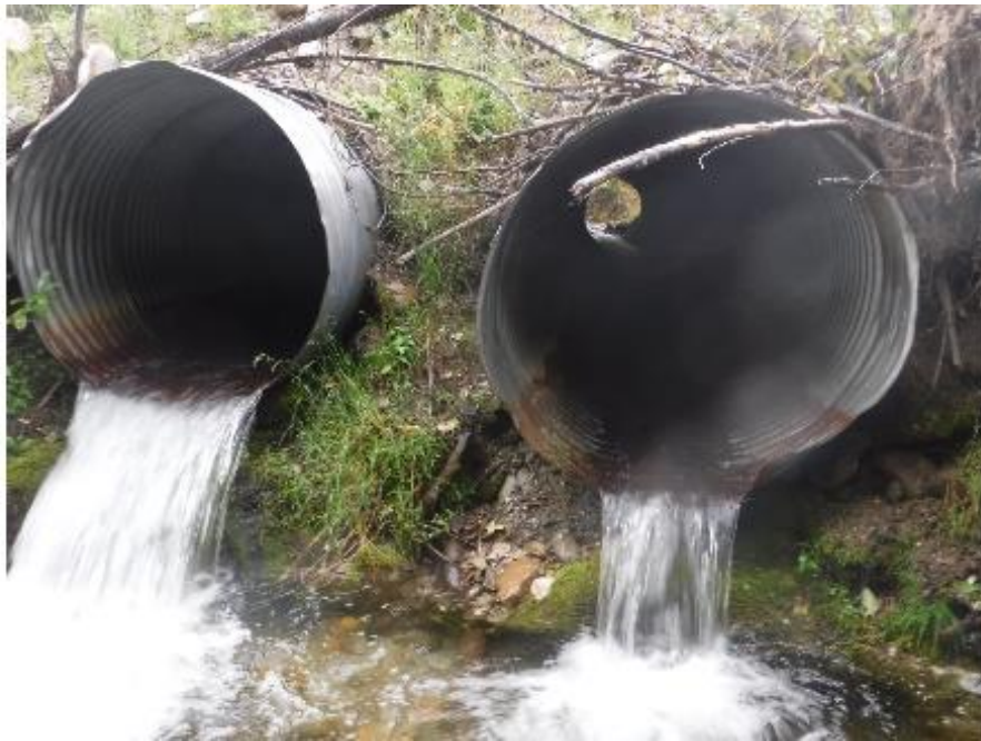
Figure 68: Outlet of PSCIS crossing 125231 (UTM: 10N 549976 6065139).
