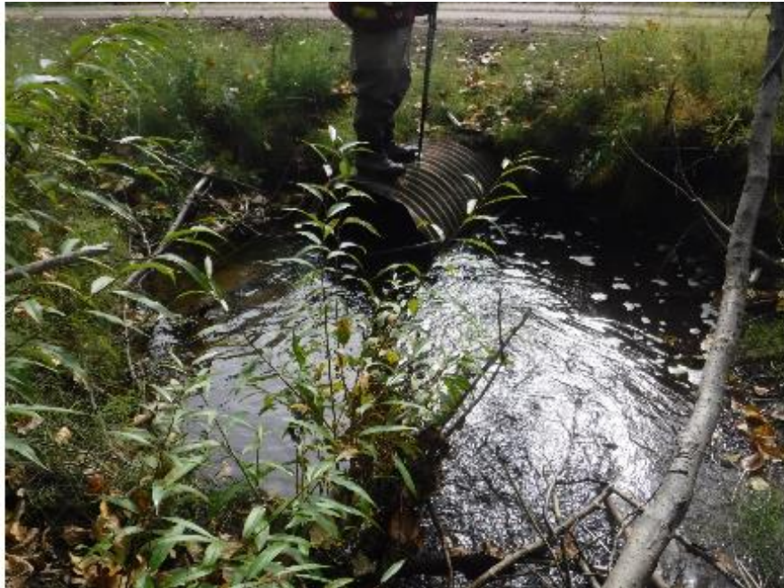
Figure 75: Inlet of PSCIS crossing 125247 (UTM: 10N 542959 6062815).
