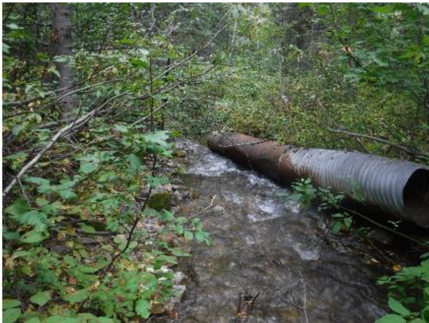
Figure 13: Corrugated culvert structure located downstream of PSCIS crossing 57690 (UTM: 10N 555118 6046103).
