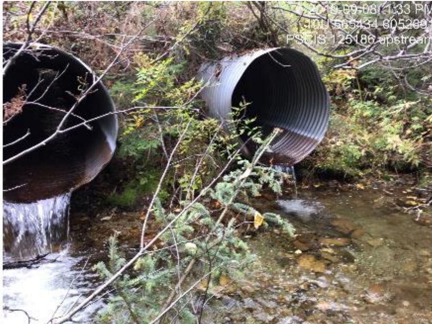
Figure 63: Inlet of PSCIS crossing 125186 (UTM: 10N 565434 6052677).
