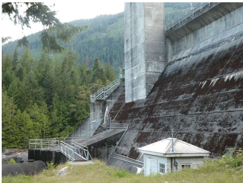
Figure 15. The Pump House at the base of the Clowhom Dam supports hundreds of bats.
