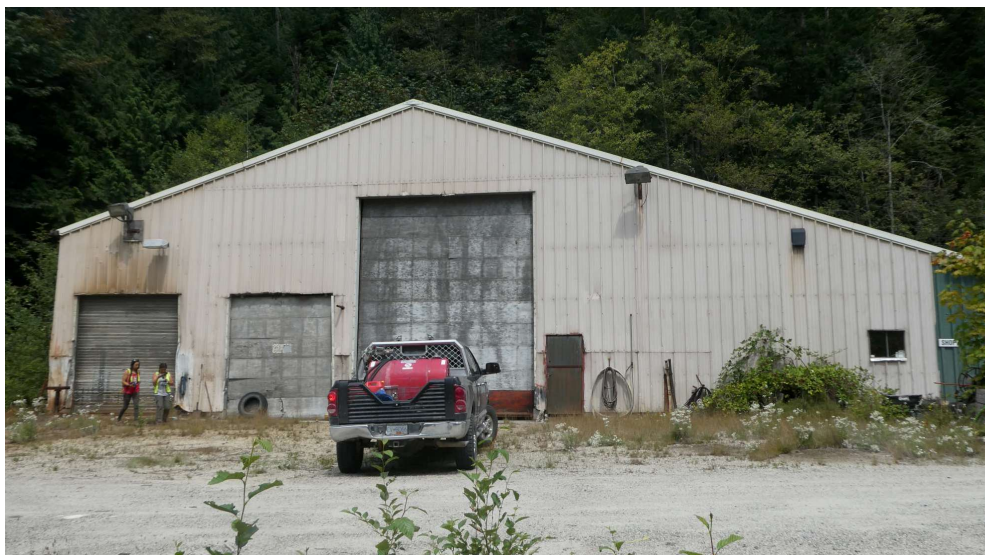
Figure 14. The Clowhom Village Warehouse contains a small bat roost.
