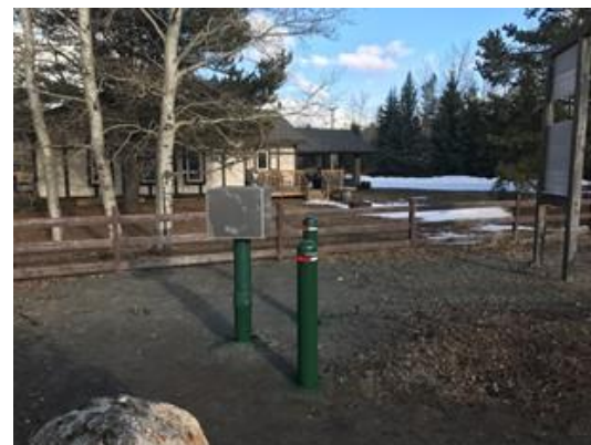
View of completed well OW502, Valemount.
