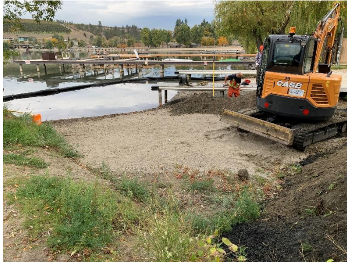
Photo 1 - Floating siltcurtain installed between project area and Kalamalka Lake
