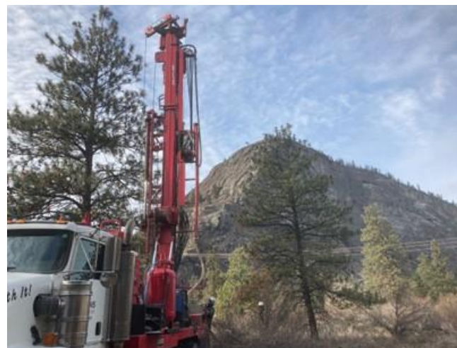
Drill rig installing OW 506 on the Vaseux Creek alluvial fan.
