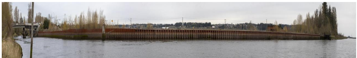
Figure 4: Panorama of the 440m steel clad retaining wall that separates the current site from Courtenay River.
