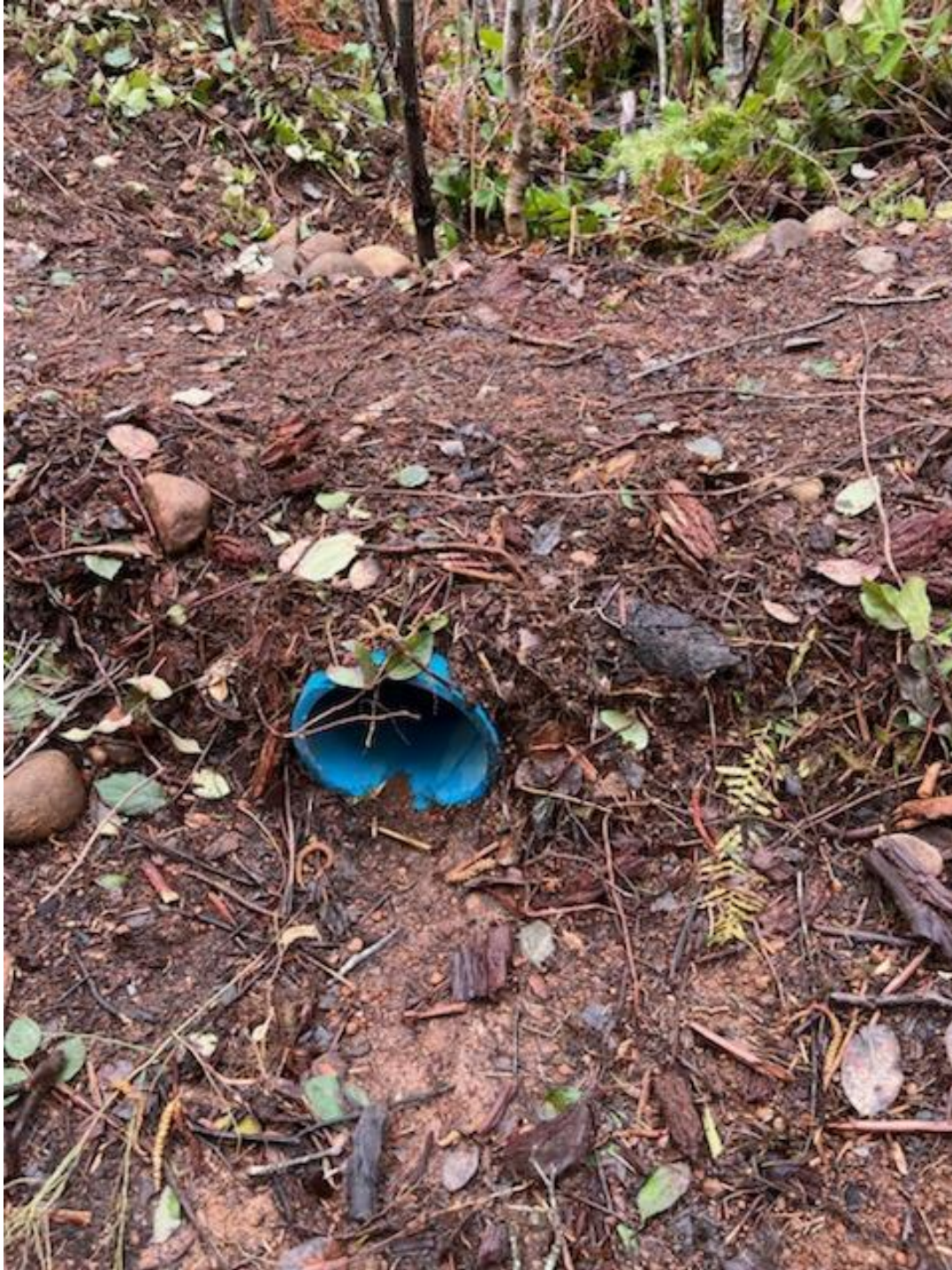
Figure 14 - PVC pipe from the work site installed for drainage in a local mountain biking trail.
