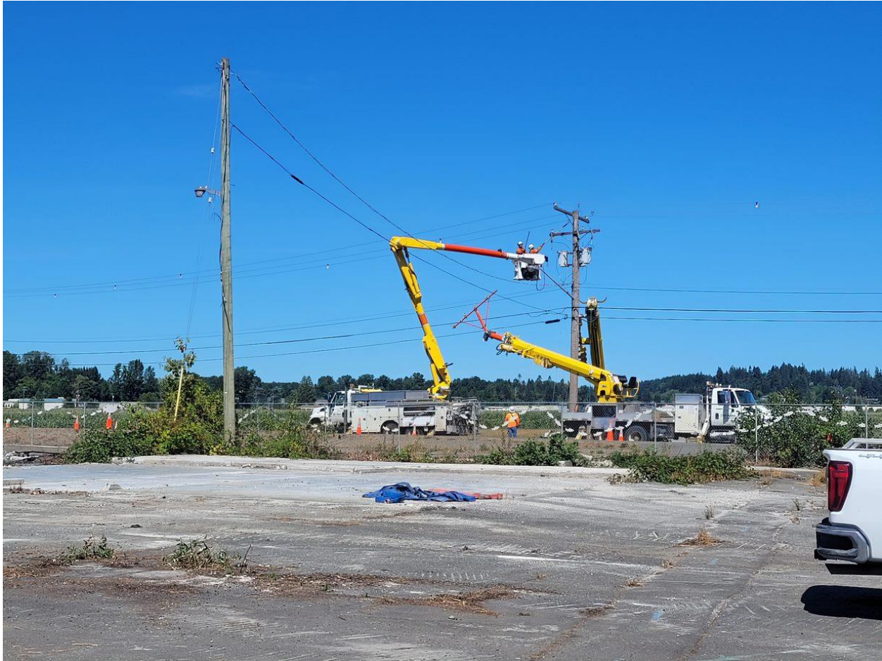
Figure 11 - BC Hydro Crew disconnecting lines to power pole at KKS site in preparation for removing it.
