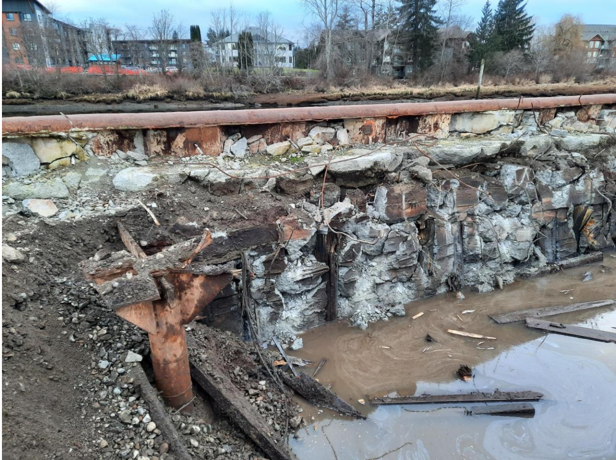
Figure 10 - Cement wall running parallel to the steel sheet piling in the process of being removed.
