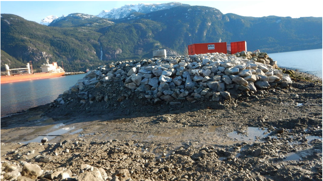
February 6, 2022. Excavation of Berm underway. Facing south towards "Spit Island".
