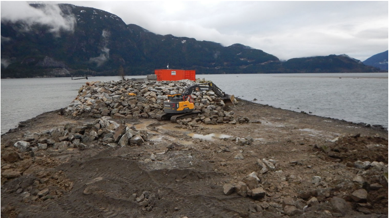
February 8, 2022. Work continues. Facing south towards “Spit Island”.
