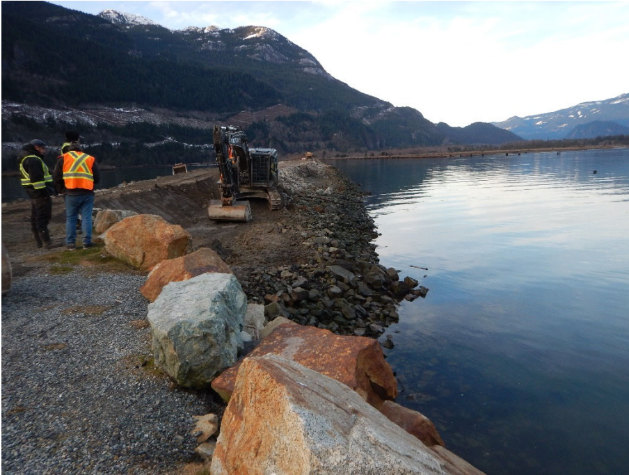
January 28, 2022. Construction commences
