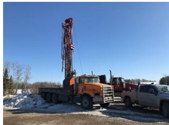
Drilling of Observation Well 516 – Vanderhoof B.C.
