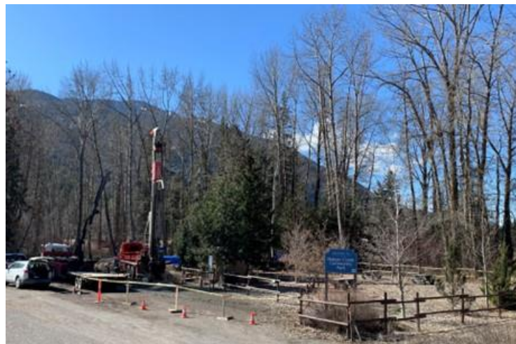
Drilling of Observation Wells 514 & 515 Photo: M. Wade
