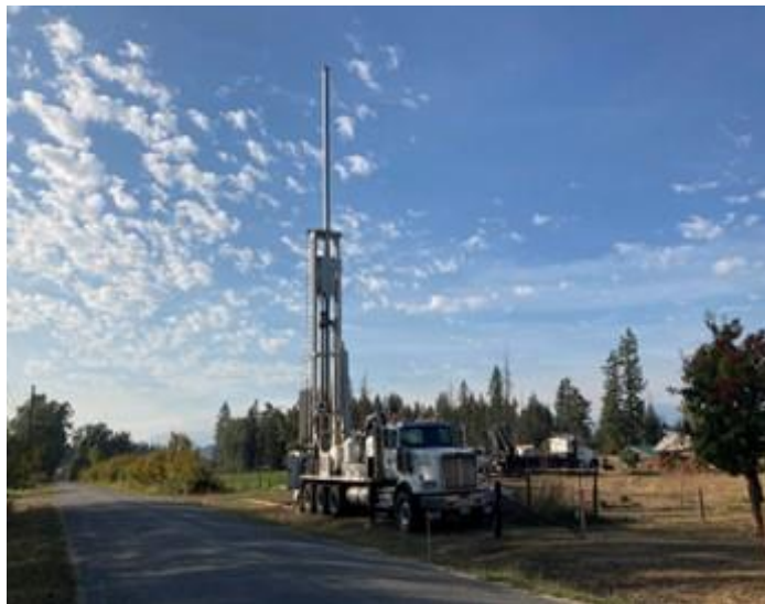
Drilling of Observation Well 509 – Canyon B.C.
