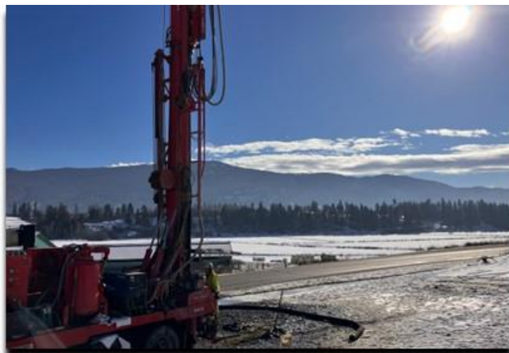
Drilling of Provincial Observation Well 510
