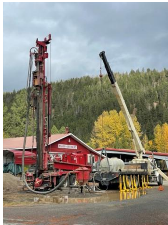
Drilling of Observation Well 508 – Tulameen B.C. Photo: J. Pogson
