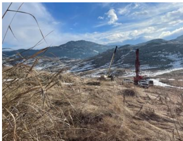
Drilling of Observation Well 512 Photo: J. Pogson
