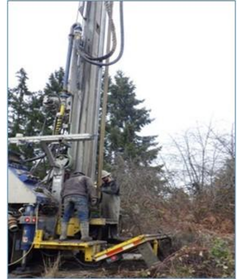
Installation of project monitoring well. Photo source: Ministry of Forests
