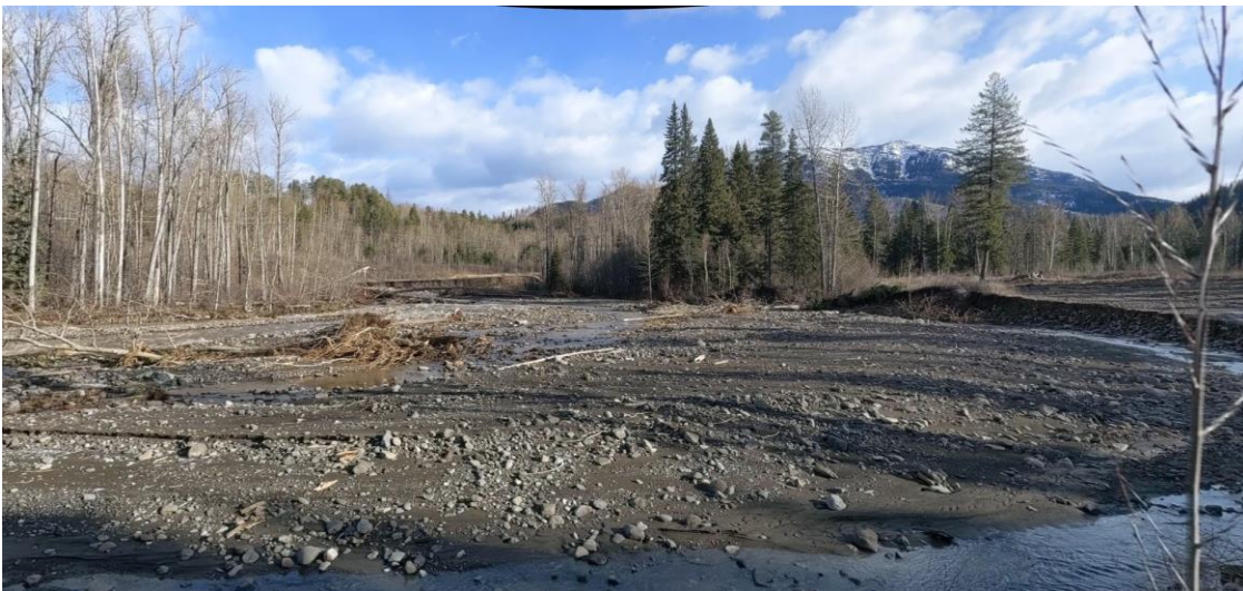
Figure 1: Flood damage to an Elk Valley watercourse (Coal Creek) during the November 2021 flood event.
