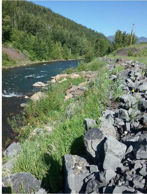
Figure 5: Example of site where rehabilitation has been determined not possible or necessary.
