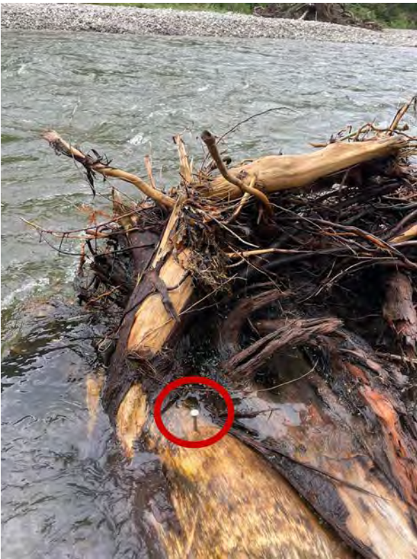
Figure 17. First W structure. Upstream key log.
