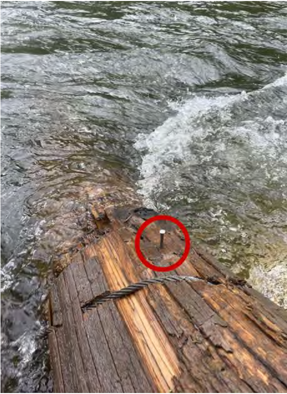
Figure 22. Third W structure. Downstream key log.
