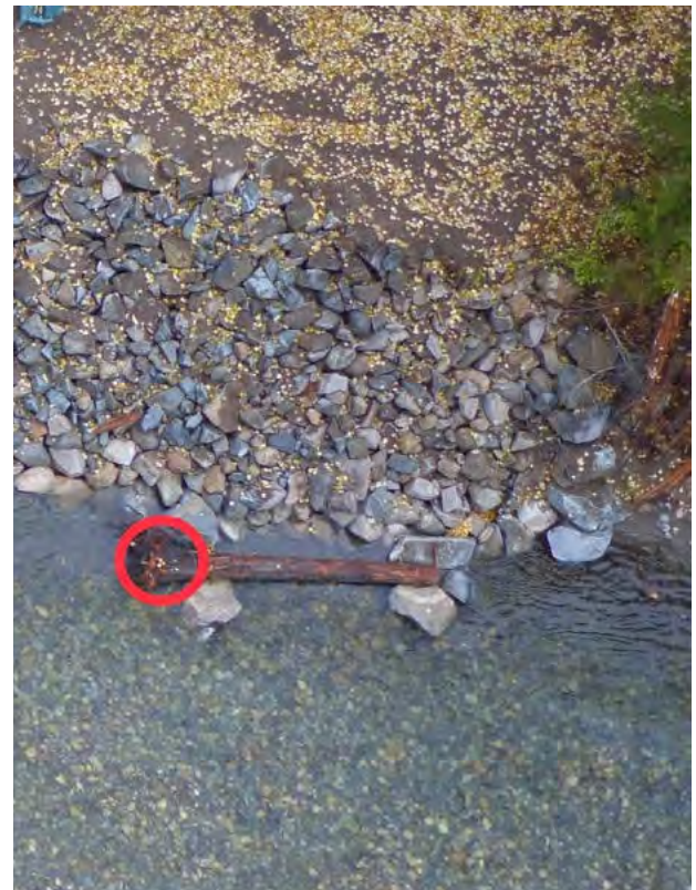
Figure 12. Benchmark for 2 upper triangles. (Not including downstream key log of second triangle. Second triangle downstream key log shares benchmark with First lateral log).
