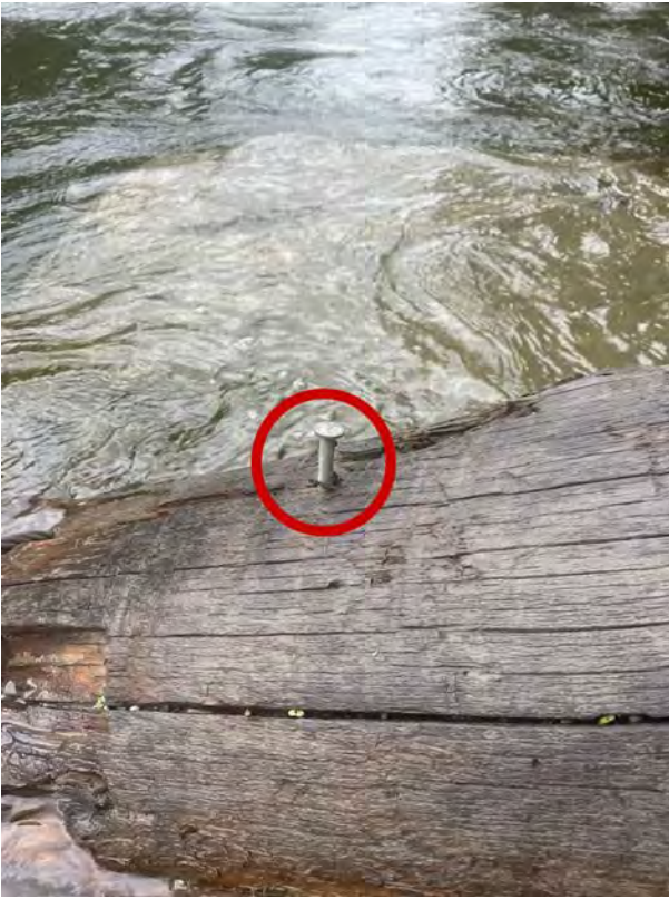
Figure 20. Second W structure. Downstream key log.
