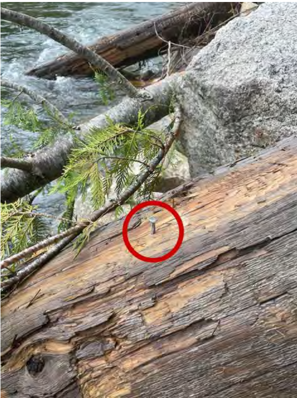
Figure 23. Fourth W structure. Upstream key log.
