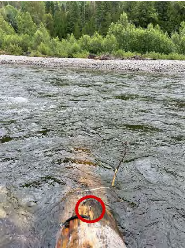
Figure 18. First W structure. Downstream key log.
