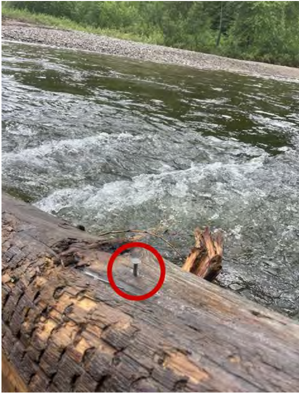
Figure 24. Fourth W structure. Downstream key log.
