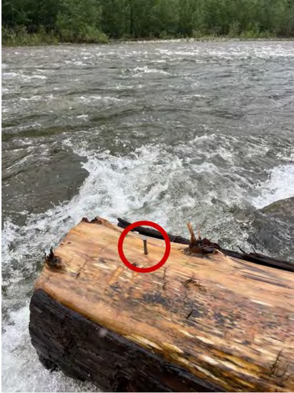
Figure 5. Debris Catcher. Downstream top log.
