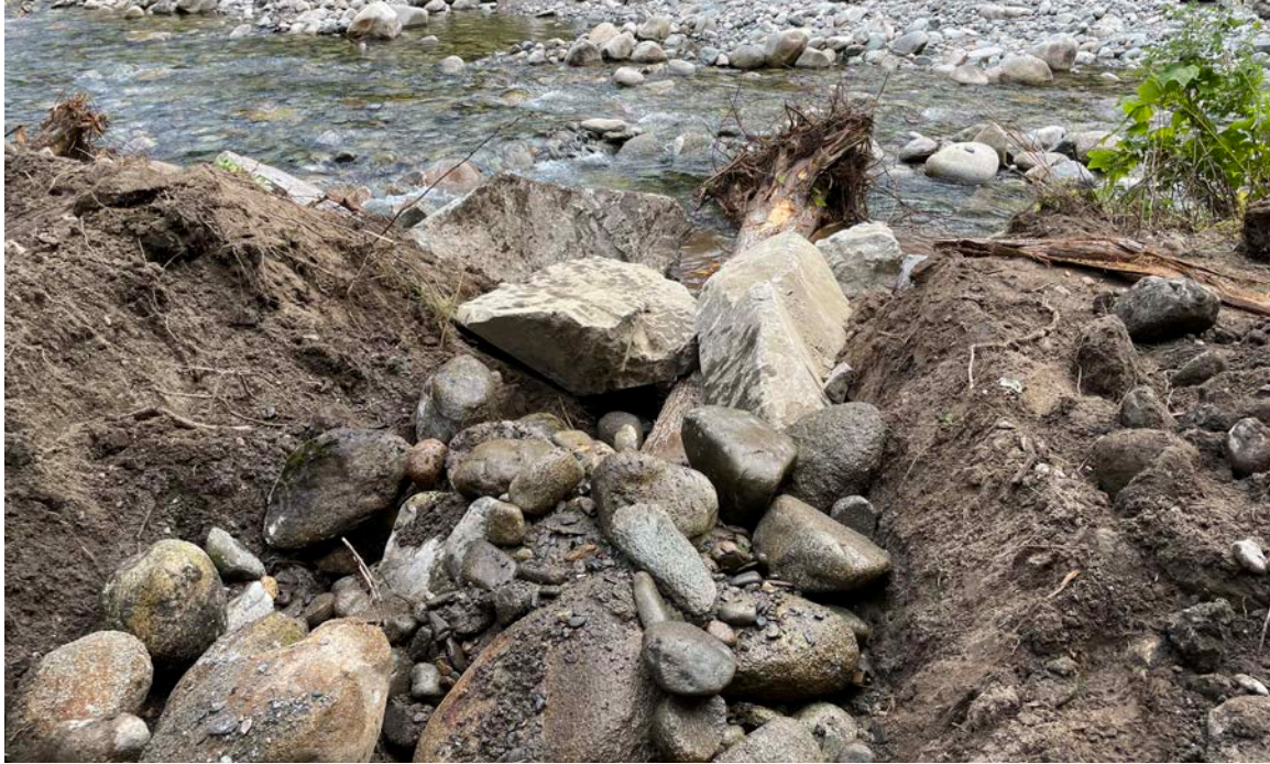
Site B: Rootwad Trenching/Ballasting: One Meter Extension into the River.
