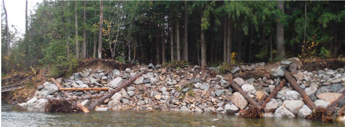
Downstream end of Site A: shows Triangular Structure C/W 2 Ramp logs and a 'W' structure
