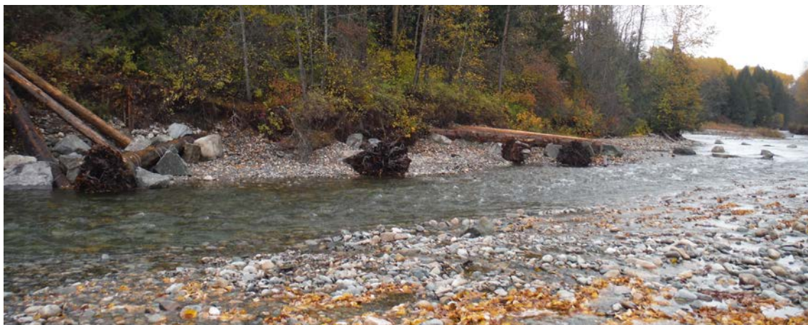
Shows upper Triangle above left, a Lateral Log structure and end view of the Debris Catcher.
