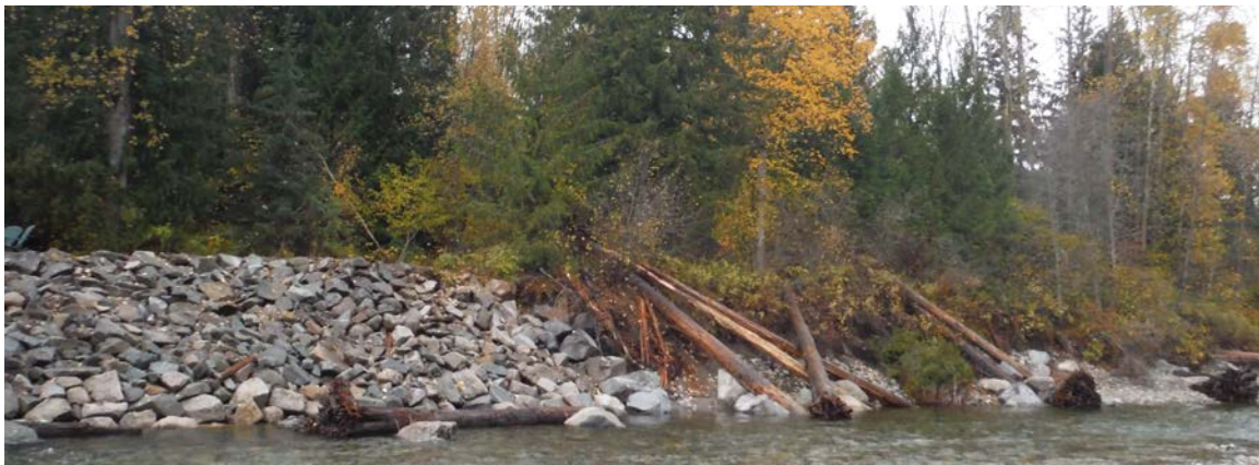
Upper end of Stabilization: Shows a Lateral Log C/W rootwad and 2 Triangular structures.
