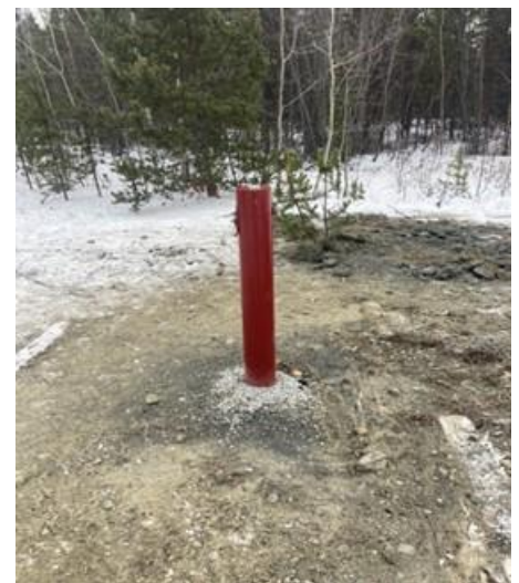
Completed monitoring well at Atlin Airport. Photo: J. Yin
