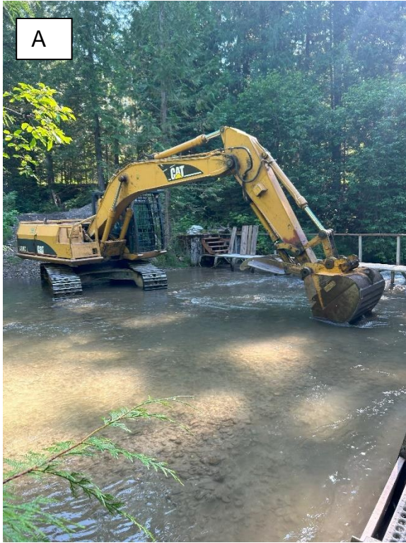
Figure 8. Main settling pond. Clearing out accumulated sediment upstream of the hatchery diversion fence (A). Bottom of main settling pond scraped clean of accumulated sediment (B).
