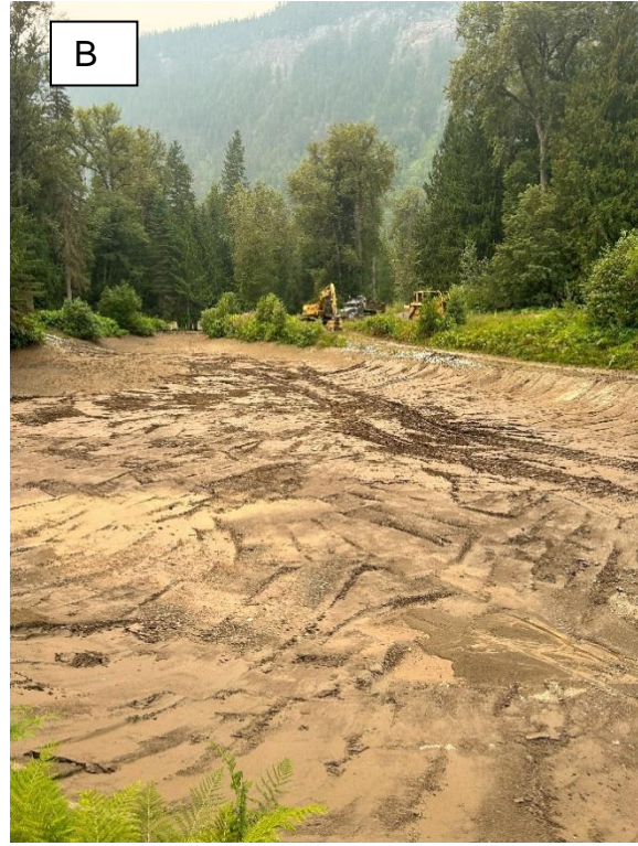
Figure 8. Main settling pond. Clearing out accumulated sediment upstream of the hatchery diversion fence (A). Bottom of main settling pond scraped clean of accumulated sediment (B).
