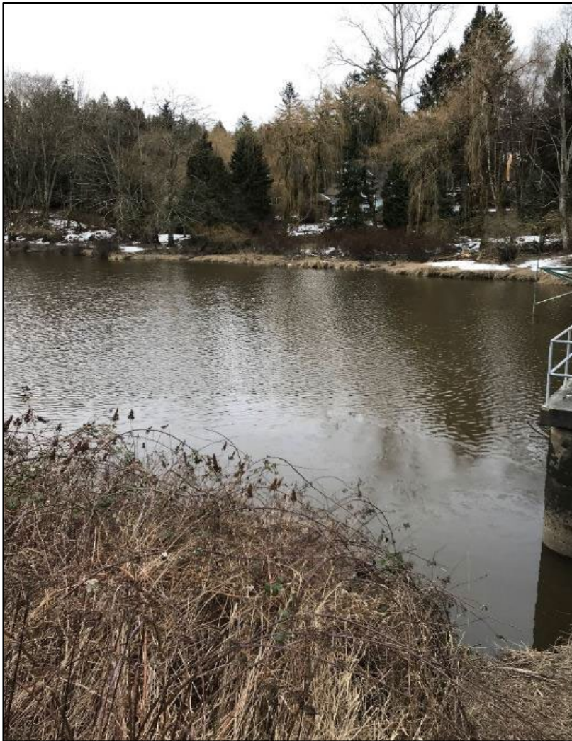
Photo 17. Looking upstream at the Nicomekl River immediately upstream of the sea dam on February 27, 2019 (near the King George Boulevard/Highway 99A bridge crossing).
