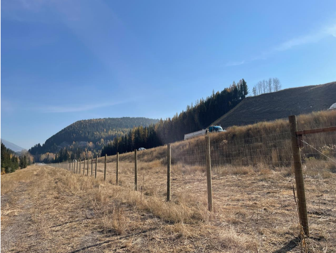
Image 6. Phase one wildlife exclusion fencing between Loop Bridge and Carbon Bridge.
