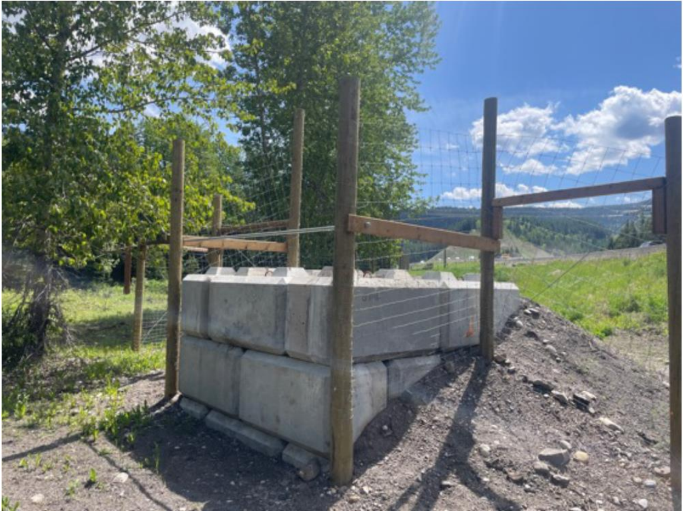
Image 7. A jumpout along the Phase one fence. The jumpout was designed based on extensive testing from Arizona using elk, bighorn sheep, and deer (Gagnon et al. 2020). This design is simple and allows animals to safely exit the highway if needed, while precluding animals from jumping into the highway right of way in reverse. Where sheep are a concern the grooves between the blocks should be filled. The horizontal bar at 45 cm above the exit ramp reduces animals jumping back into the right of way.
