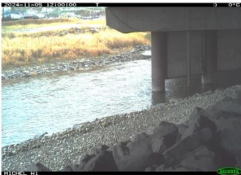
Image 4. Example of an underpass retrofit at Michel Mouth Bridge. A similar approach to Alexander Creek was used here, where a 1.5 m wide path was created through the large rip rap and filled with pea gravel to create a surface more amenable to wildlife use on both sides of the bridge.
