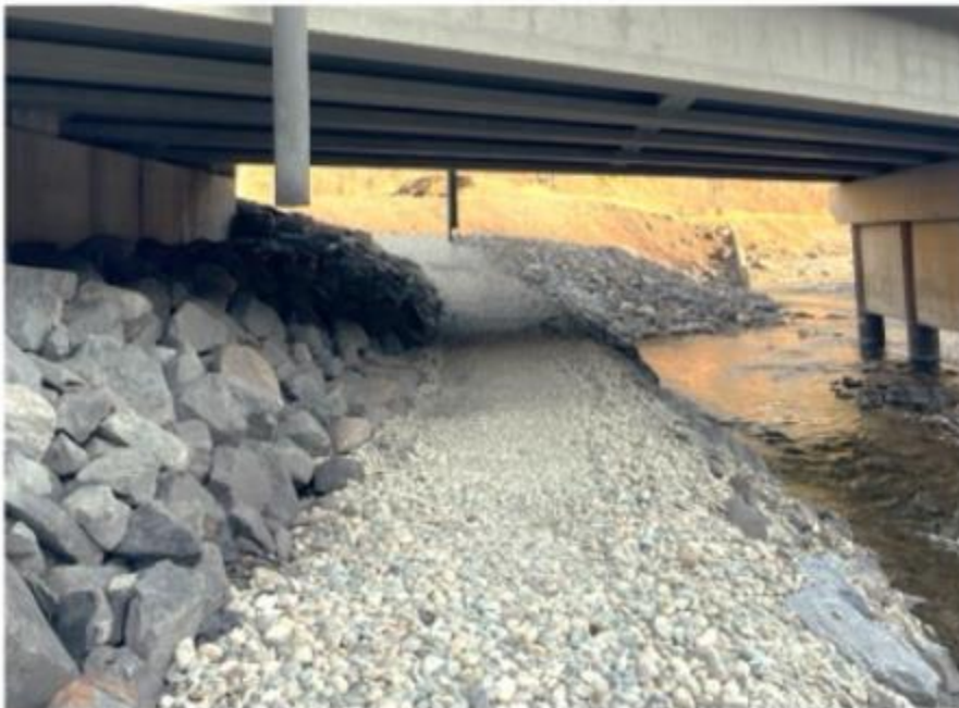
Image 5. Example of an underpass retrofit at Old Town. A similar approach to Alexander Creek was used on the NW side of the bridge, where a 1.5 m wide path was created through the large rip rap and filled with pea gravel to create a surface more amenable to wildlife. The SE side of the bridge was already very open and serving as an underpass with no work needed.
