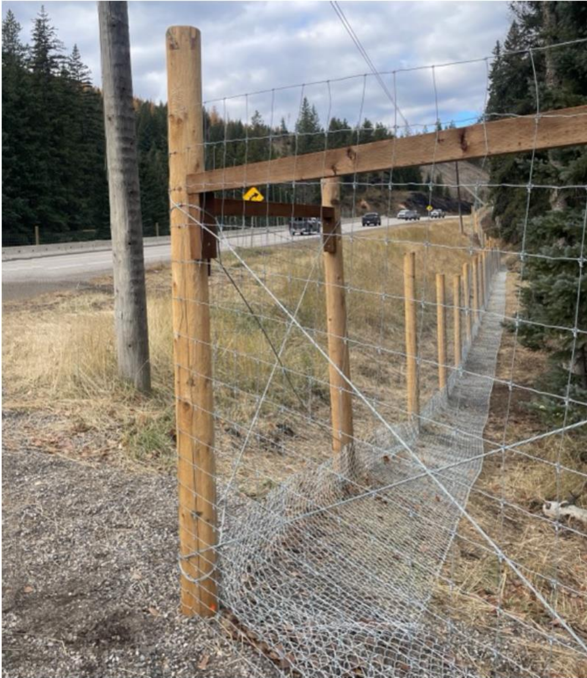
Image 8. Phase two wildlife exclusion fencing between Carbon Bridge and Alexander Bridge. Chain link skirting to reduce animals digging under the fence shown at the bottom.
