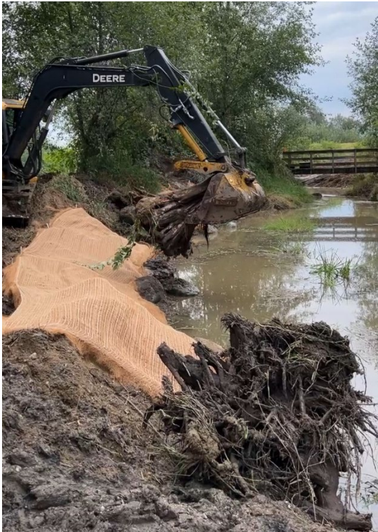
Figure 12 Large woody debris installation
