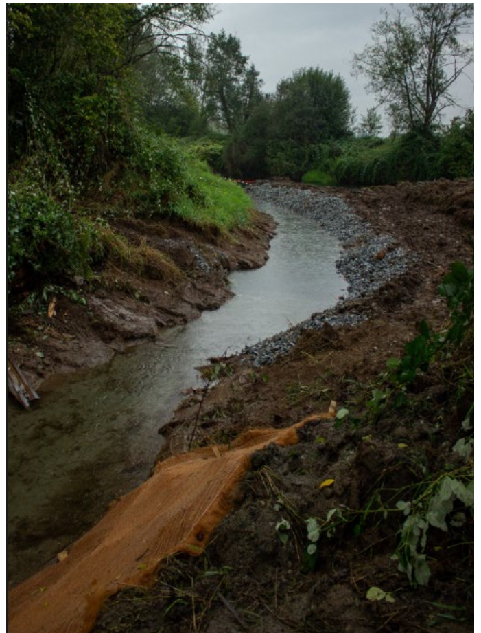
Figure 11 Upstream portion - Before and after with angular gravel and coconut matting for bank stability
