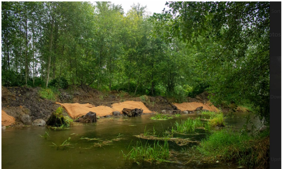
Figure 9 Pond section of Trethewey Channel with burlap coconut matting
