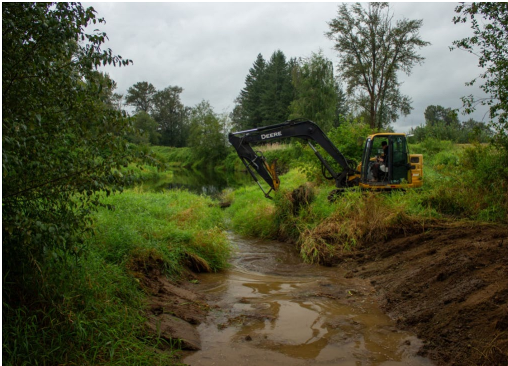
Figure 7 After - Longreach excavator in Trethewey Channel
