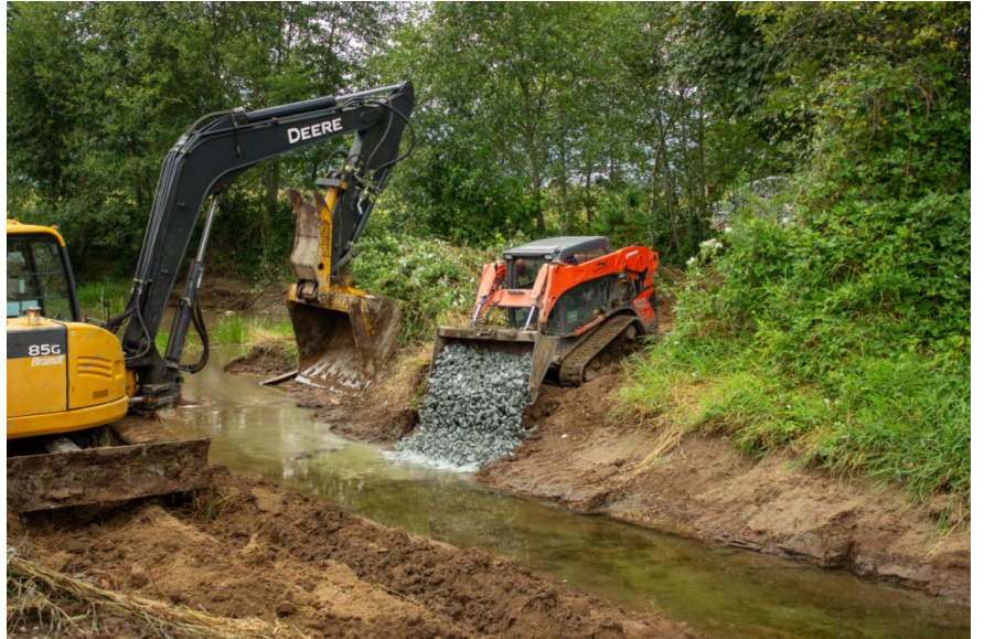
Figure 10 Addition of angular gravel on streambank
