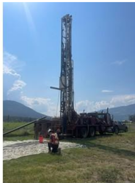
Drilling of Observation Well 518. Photo: Ministry of WLRs.
