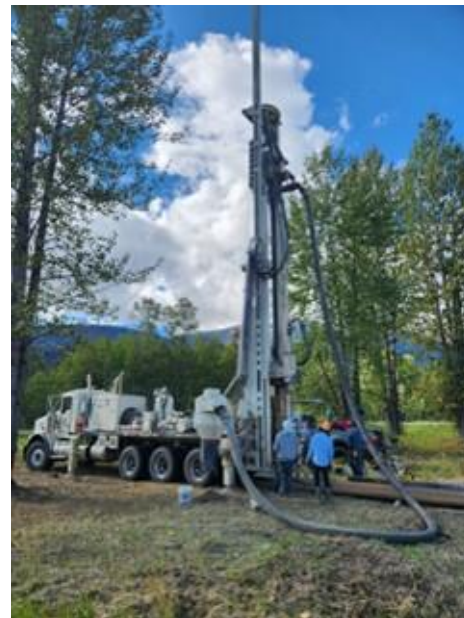
Drilling of Observation Well 520. Photo: Ministry of ENV.
