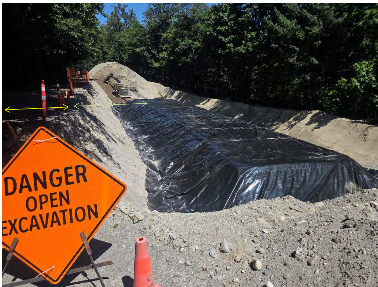
Photo 3. Placement of impervious liner covering entire JK soil complete.
