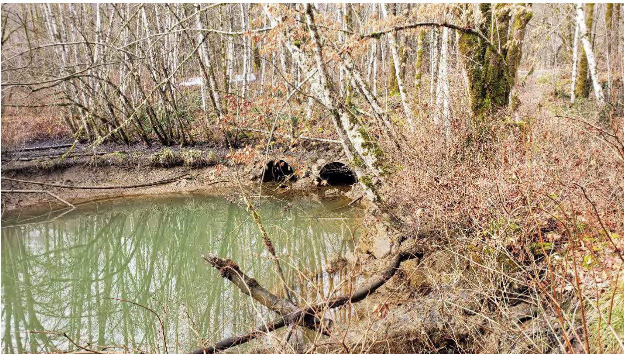
East side facing towards Training Berm and twin culvert
