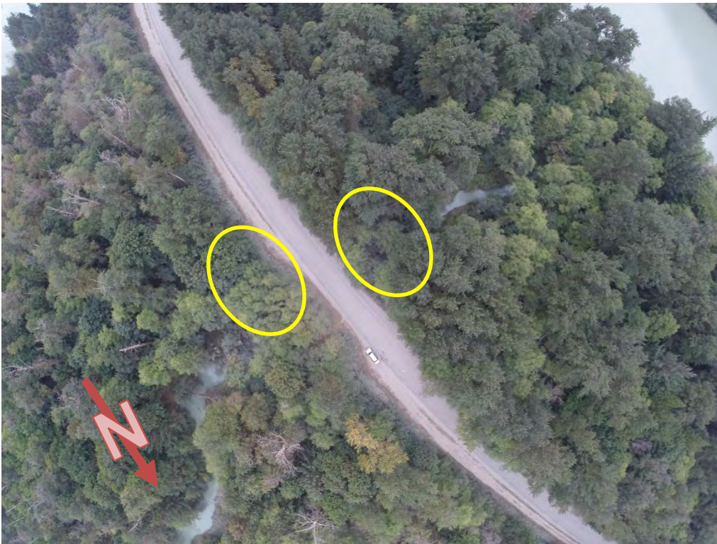
Drone overflight of culvert August 2017 (river is on right, estuary on left, and top is facing south)
