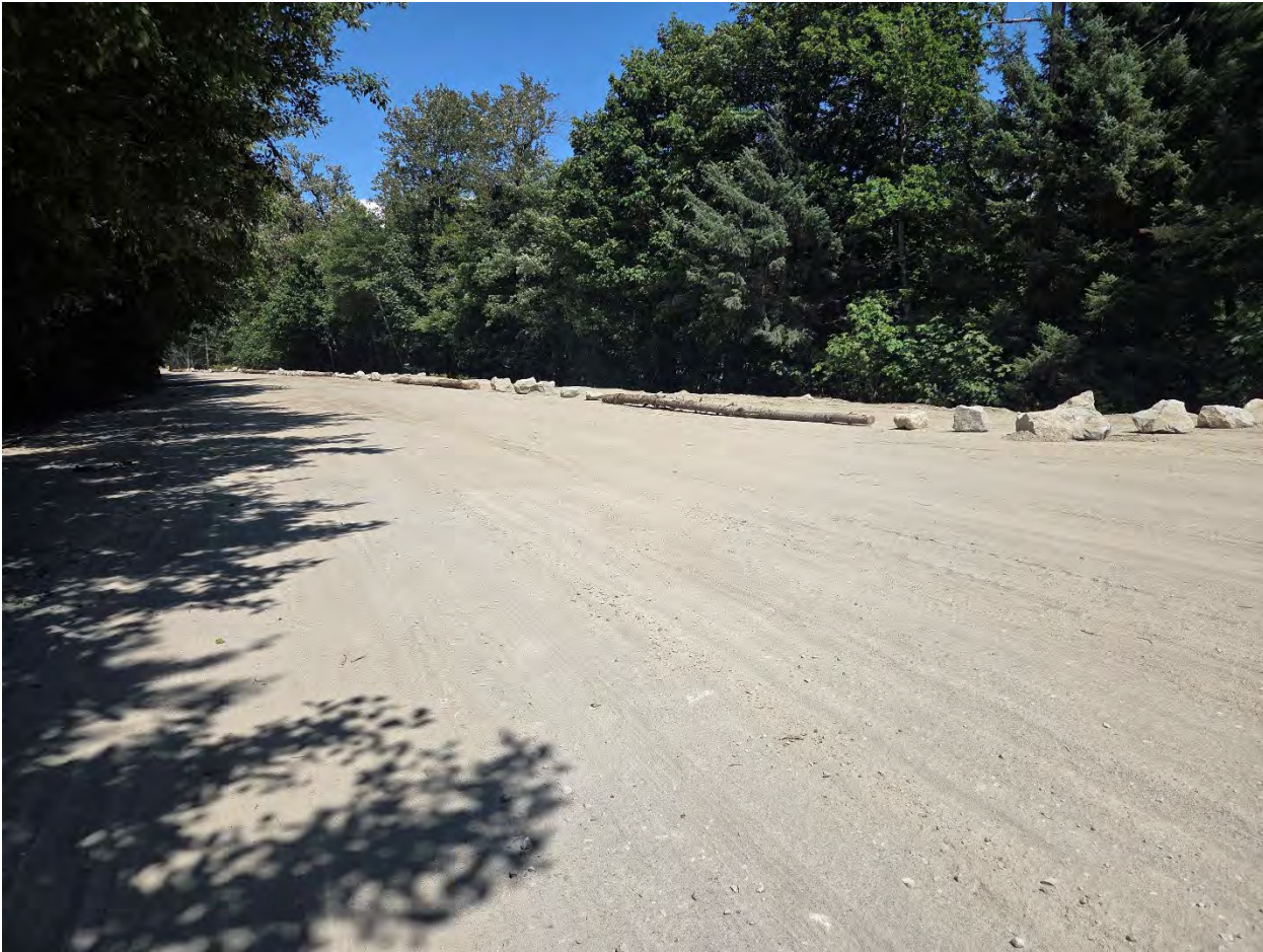
Photo 5. Road restored to original grade and compacted. Cordon of logs/rocks to prevent public from driving or parking along the shoulder and potential disturbance or distribution of knotweed.
