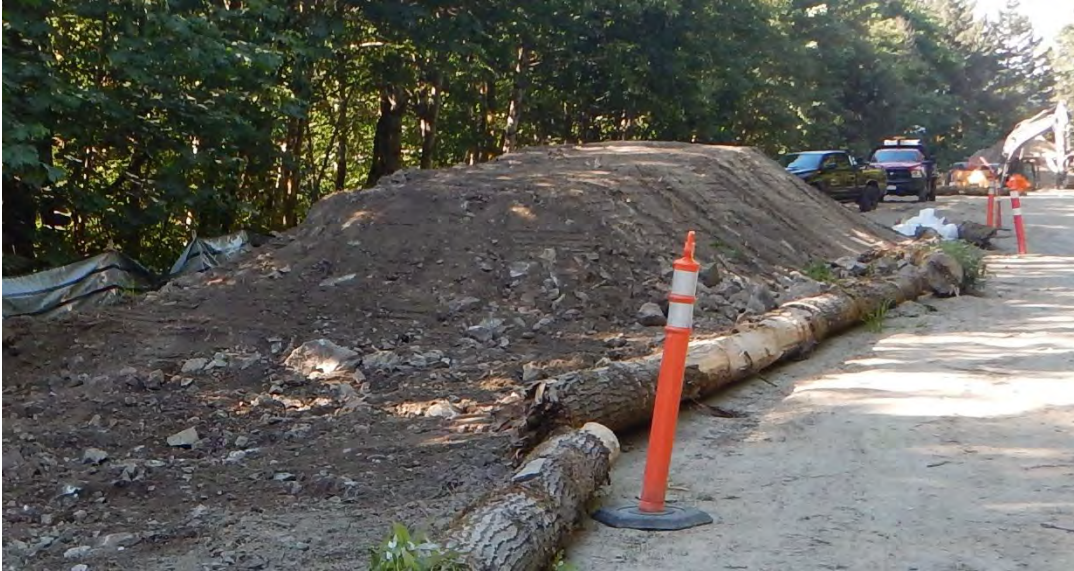
Stockpile of material from shoulder of road
