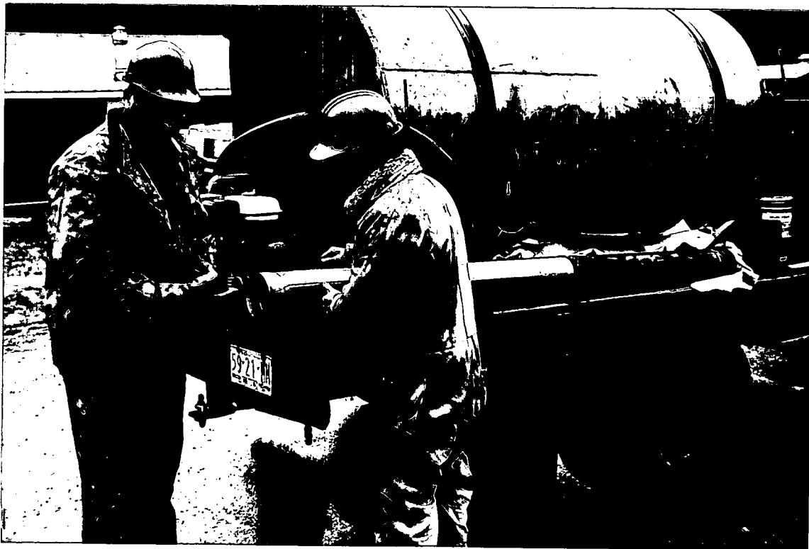
Preparing the well screen
