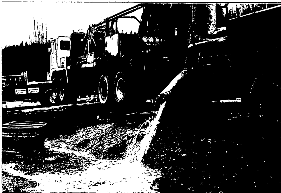
Developing the well
