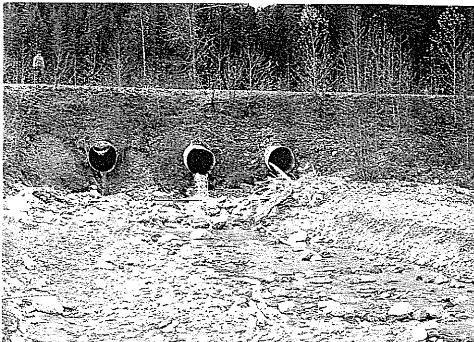
Photo 7. Culverts on Fraser Creek.
