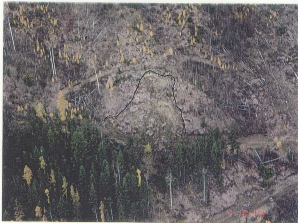
Photo 12. FE8, TP23. Large slump in fine grained soils. No sediment transfer below lower road. Road is blocked by the toe of the slide.
