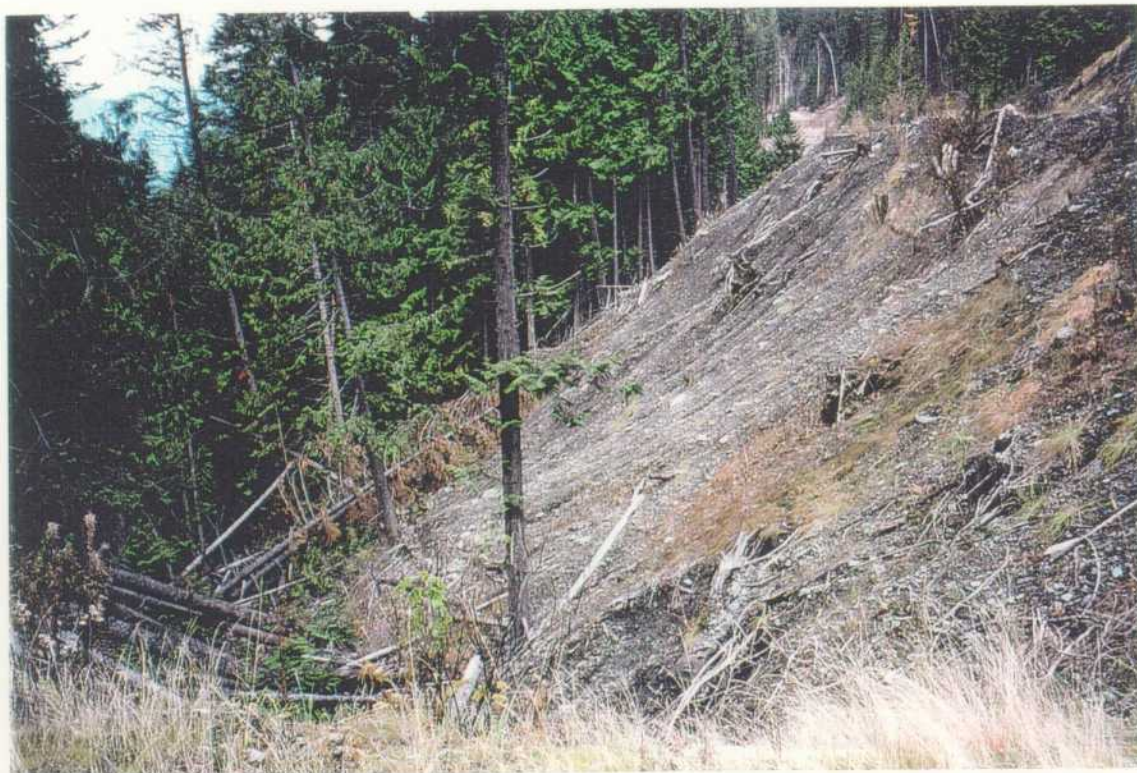
Photo 9. FE4. Failed fillslope into a gully connected to Reach 7 of Ferry Creek. Near TP11.
