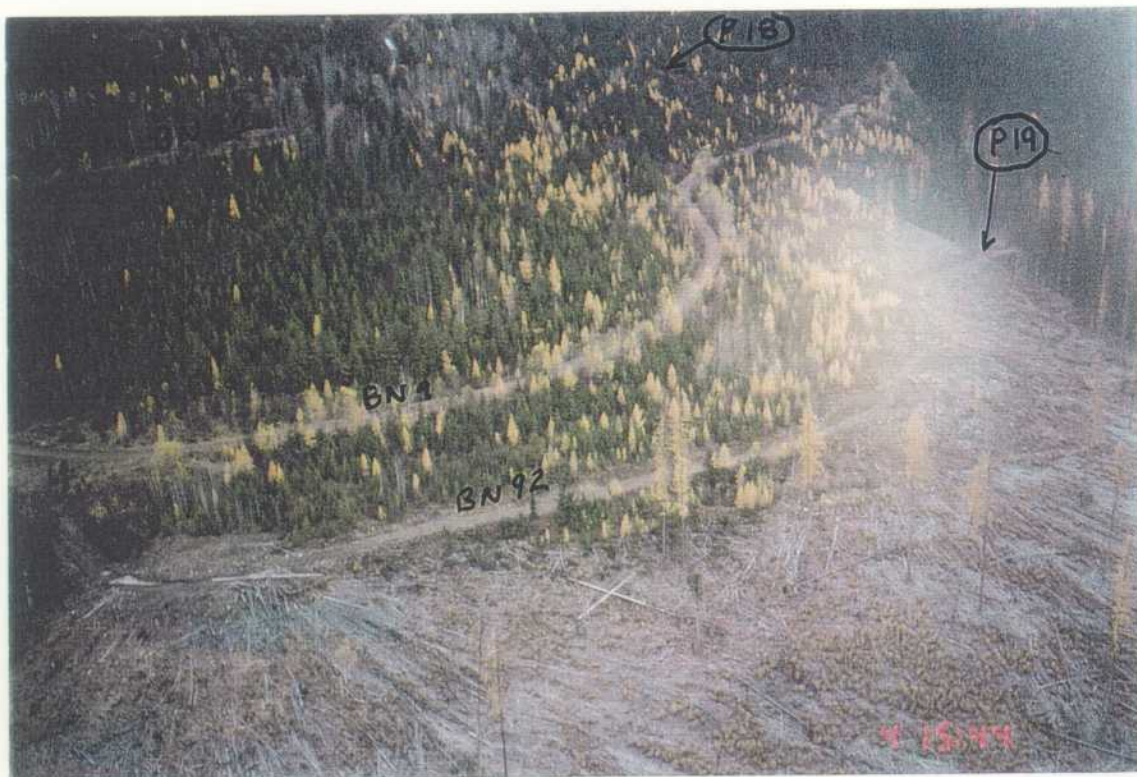
Photo 17. BN9. Road alignments on moderately steep (30 to 50%) slopes. Little sediment movement to perennial streams.
