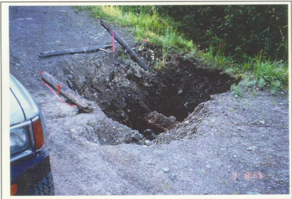
Failed wood culvert on road
