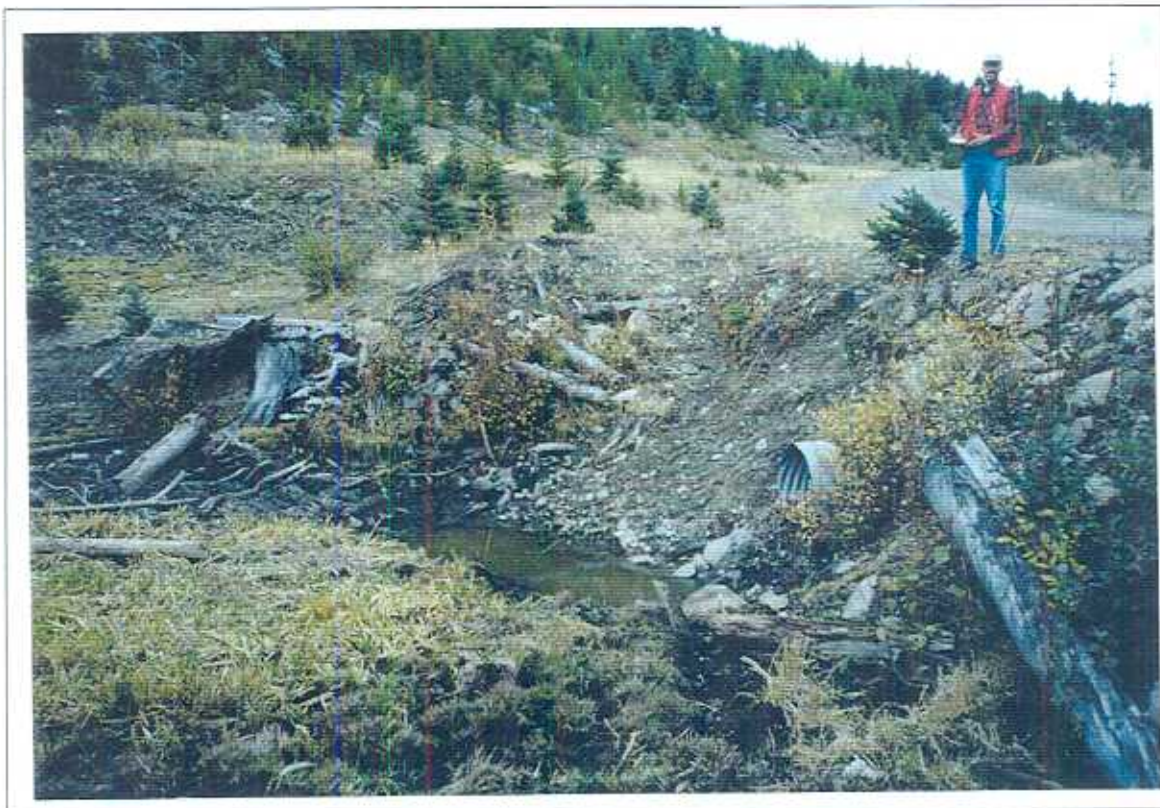
Plate 3: Sediment Source 1 - 16. km China Creek Road.
