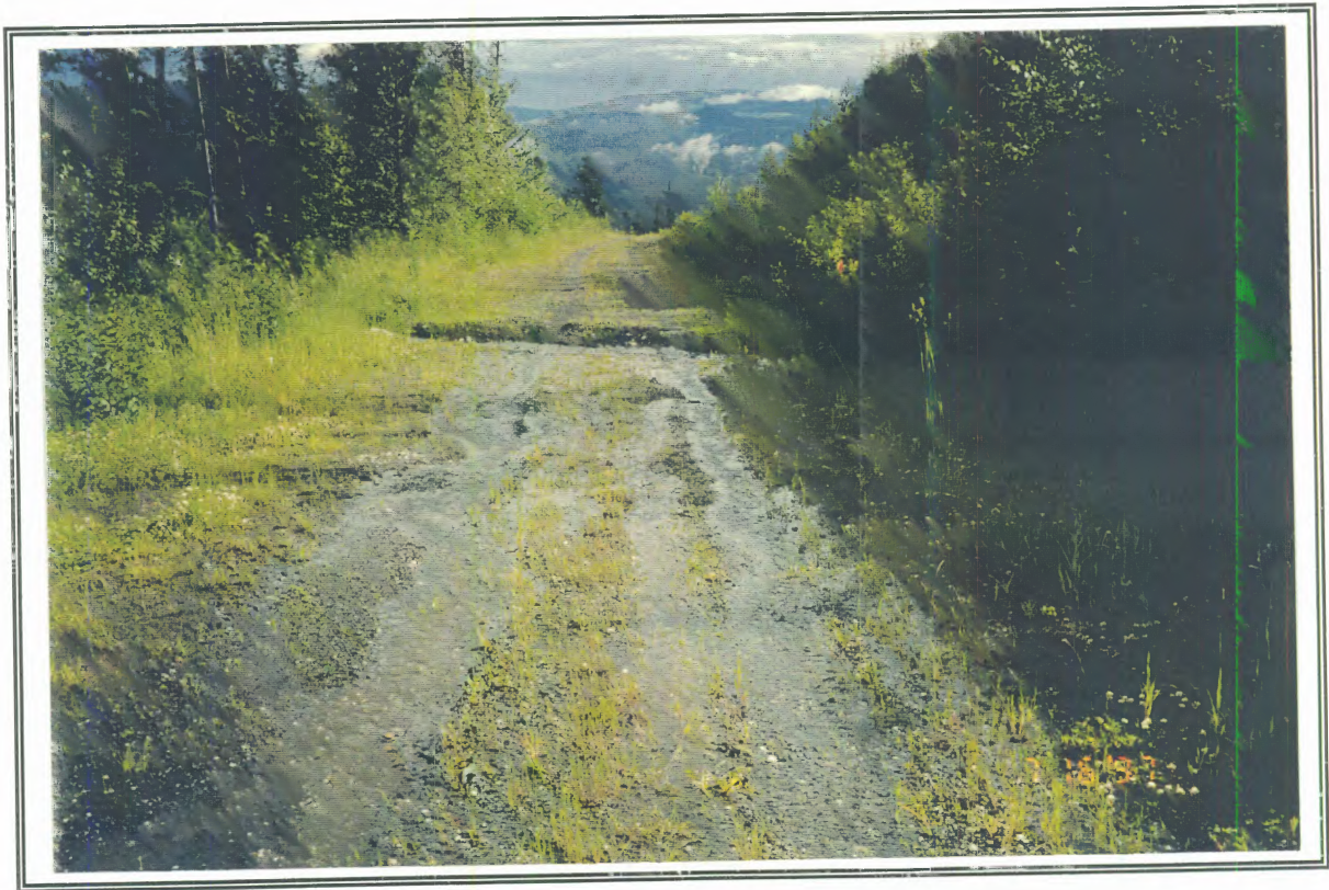
PHOTO MCKUS4. Semi-permanent deactivation on road in second major northern tributary downstream of Crooked Lake [ Site McKus3 ].
